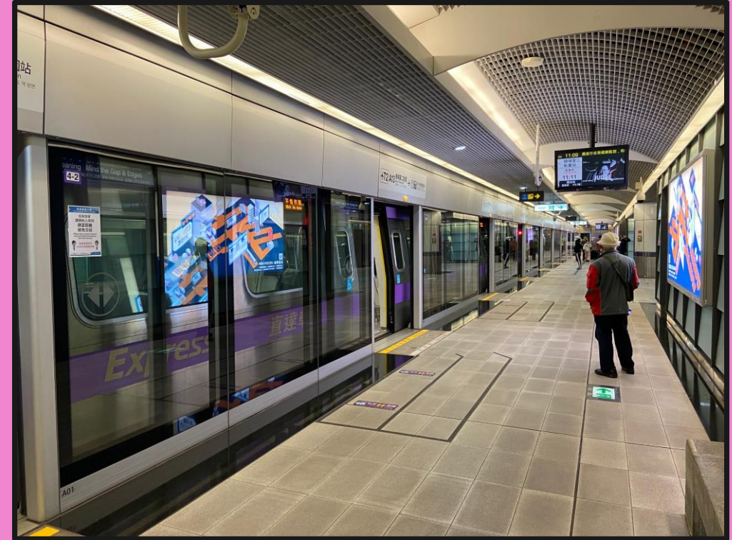
Platform screen doors currently in Taoyuan, Taiwan.
