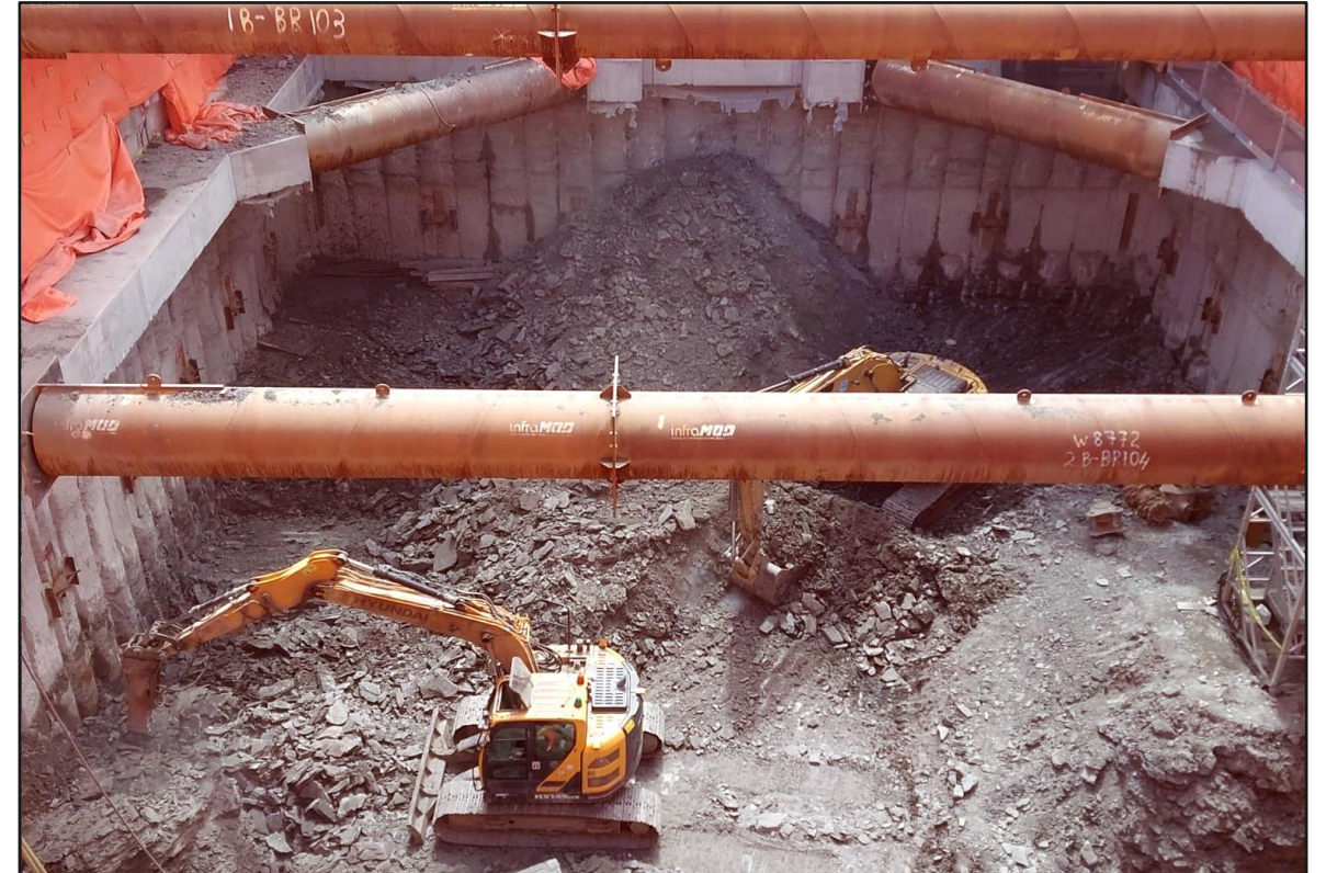
South shaft excavation looking north
