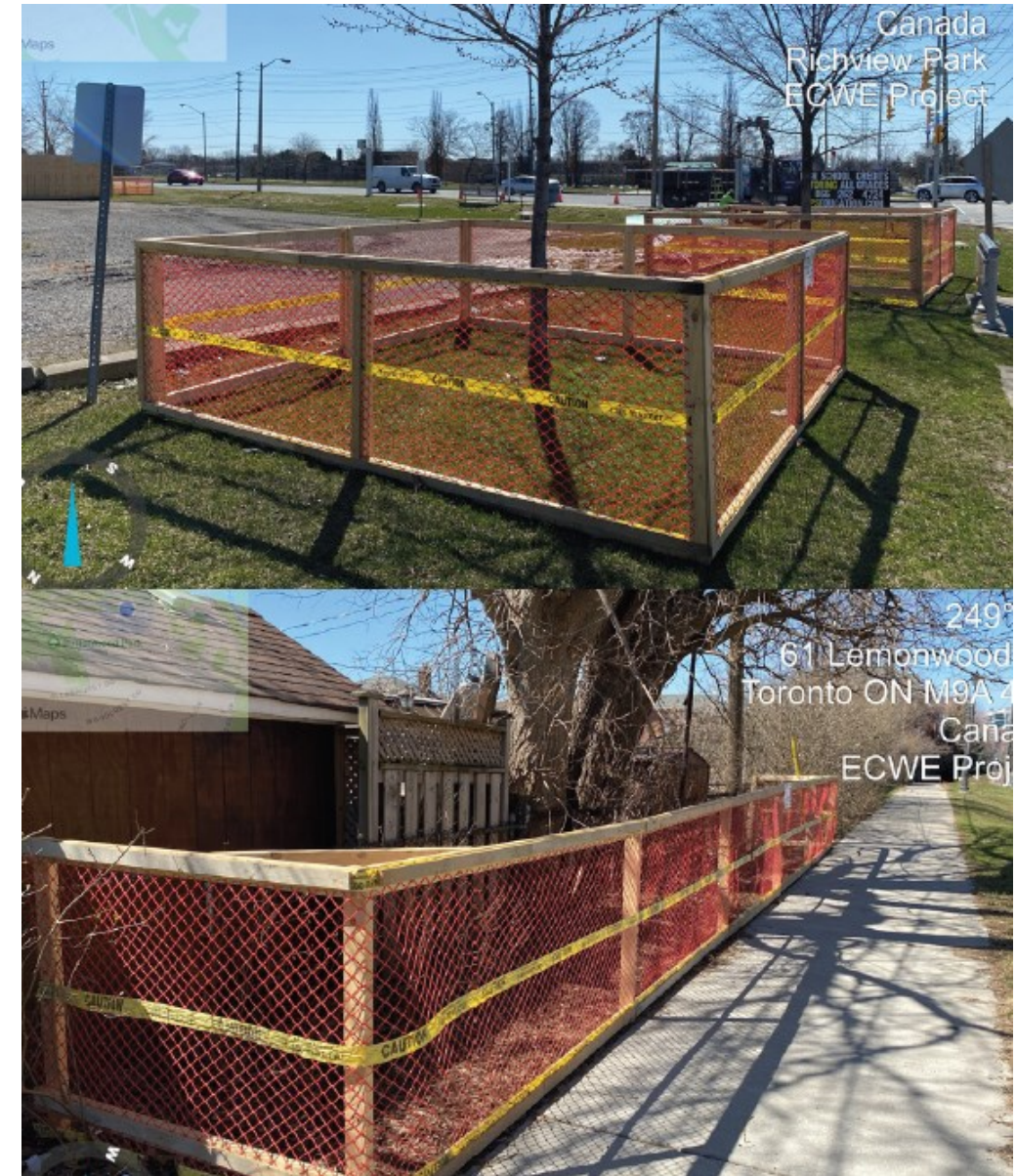
Fencing is installed around trees near construction sites to provide protection from construction activities.
