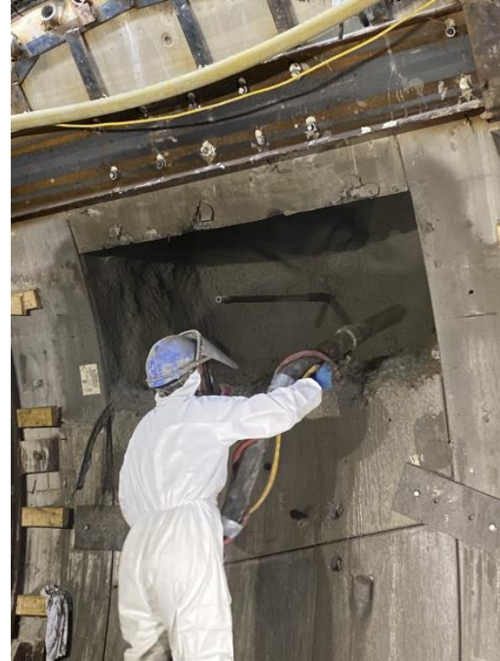
Excavation and Primary Lining
