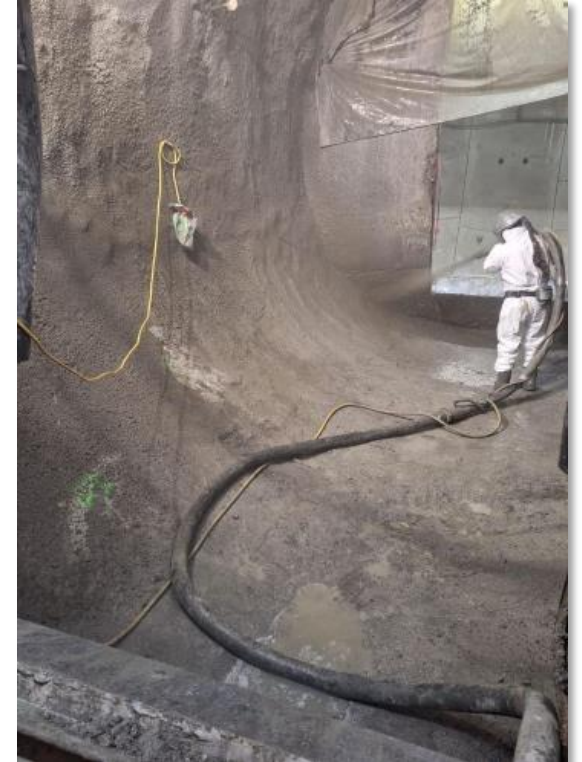
Excavation and Primary Lining
