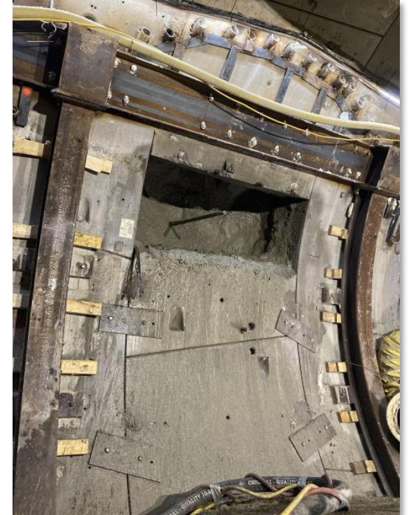
Excavation and Primary Lining
