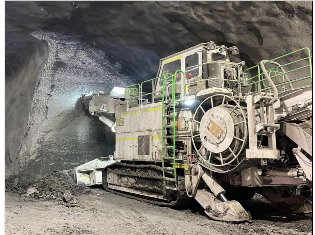
Roadheader machine removing rock to create the cavern at the future Queen-Spadina station site.
