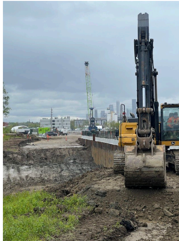
Crews working at the OMSF to construct a retaining wall to support the main building.
