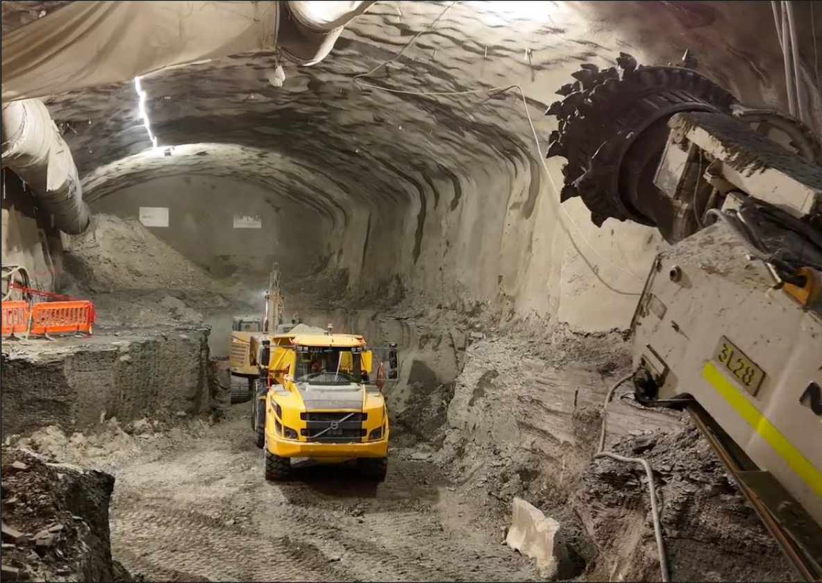
Roadheader machine removing rock to create the cavern at the future Queen-Spadina station site.
