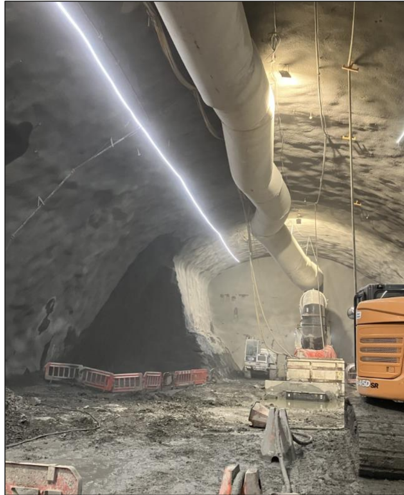
Cavern views looking at the south (left) and north (right) headwalls, with ventilation and excavation equipment on hand.
