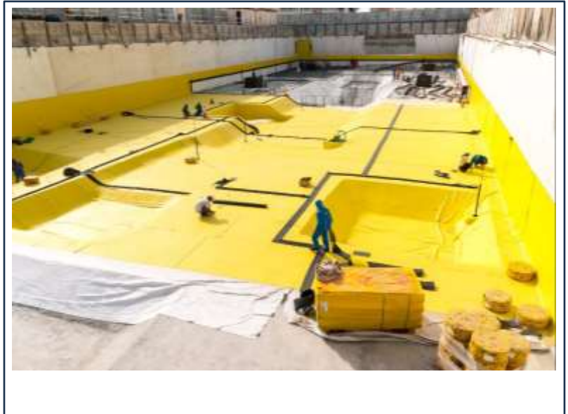
Example of waterproofing system installation
