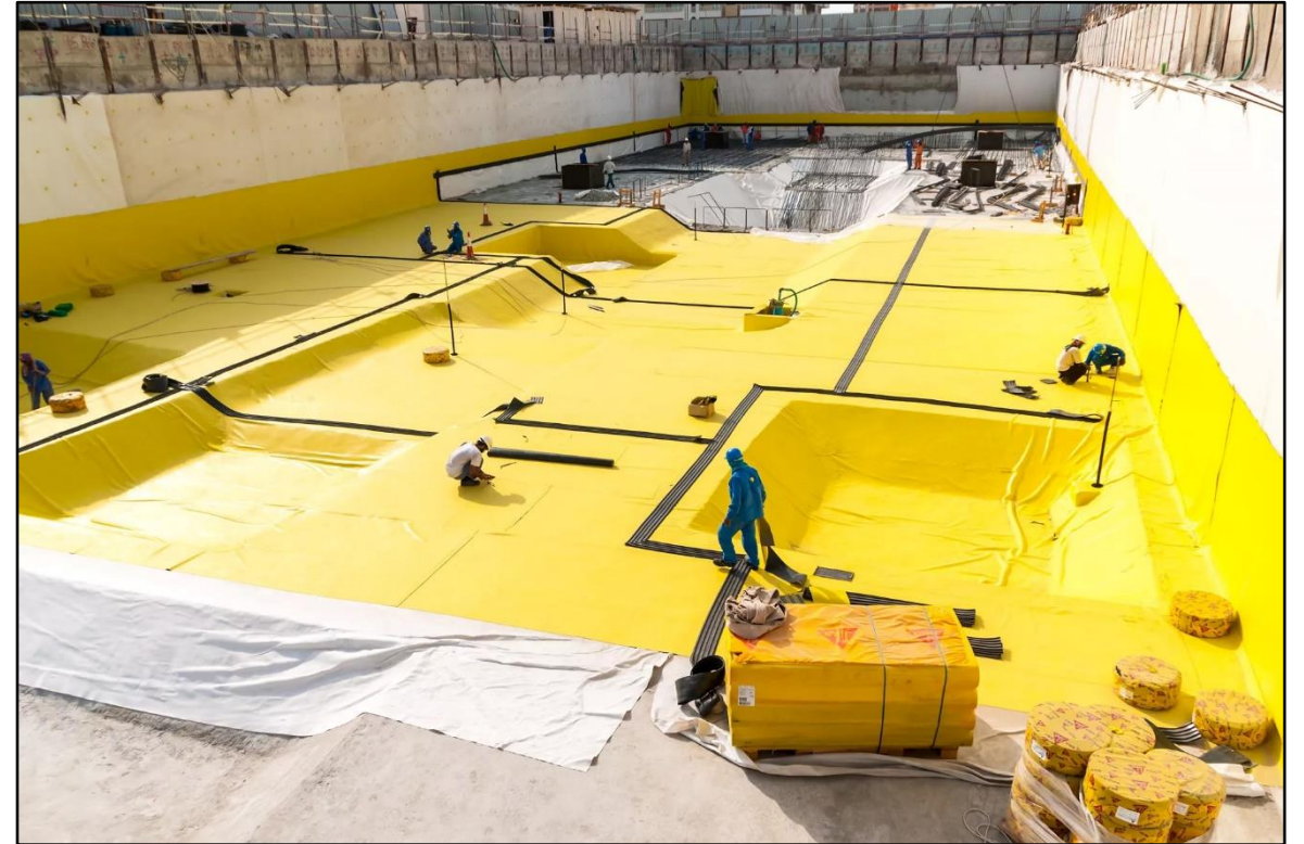
Example of waterproofing system installation
