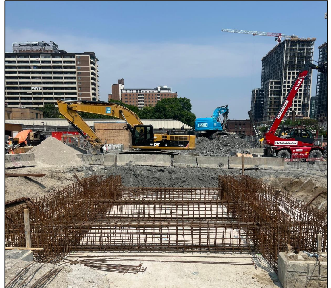
The tower crane platform foundation in progress looking north
