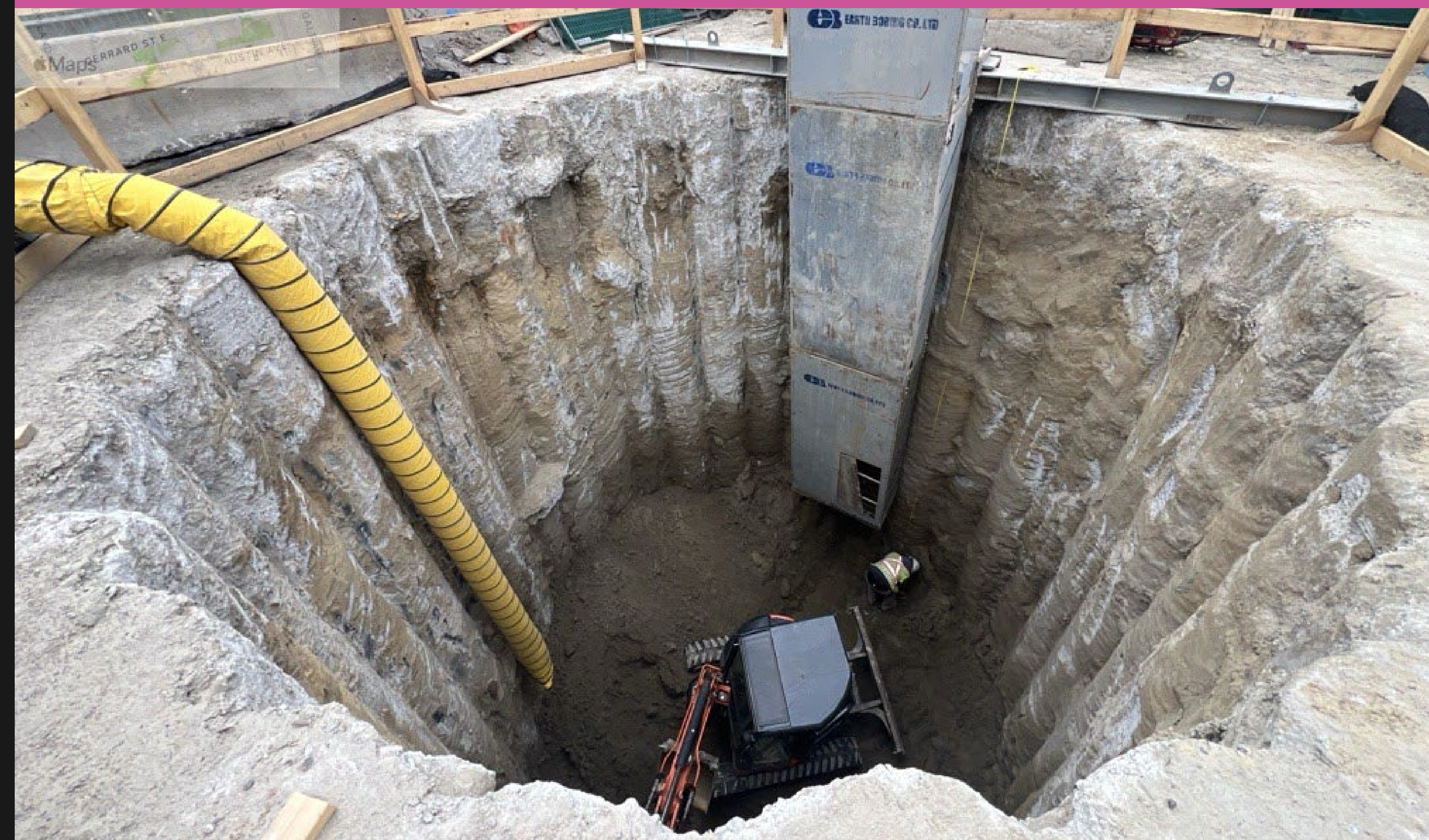
Excavation for microtunnel storm sewer launch shaft
