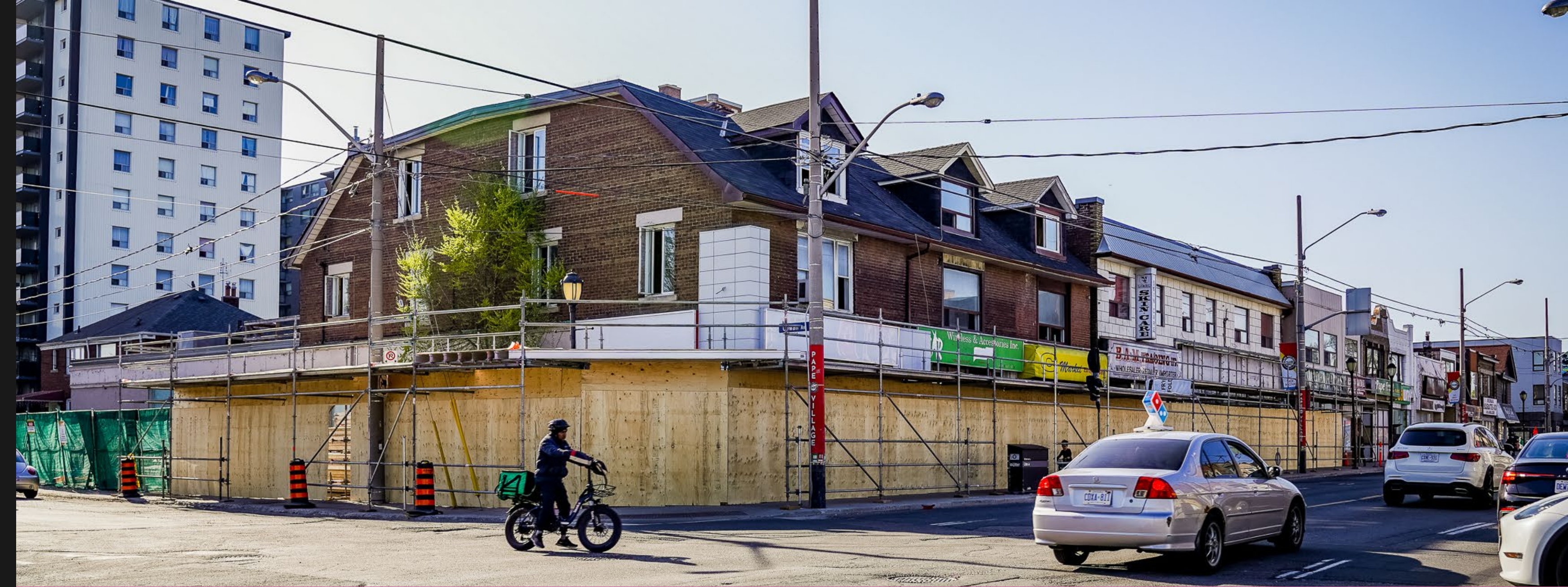
Overhead protection at Cosburn Station
