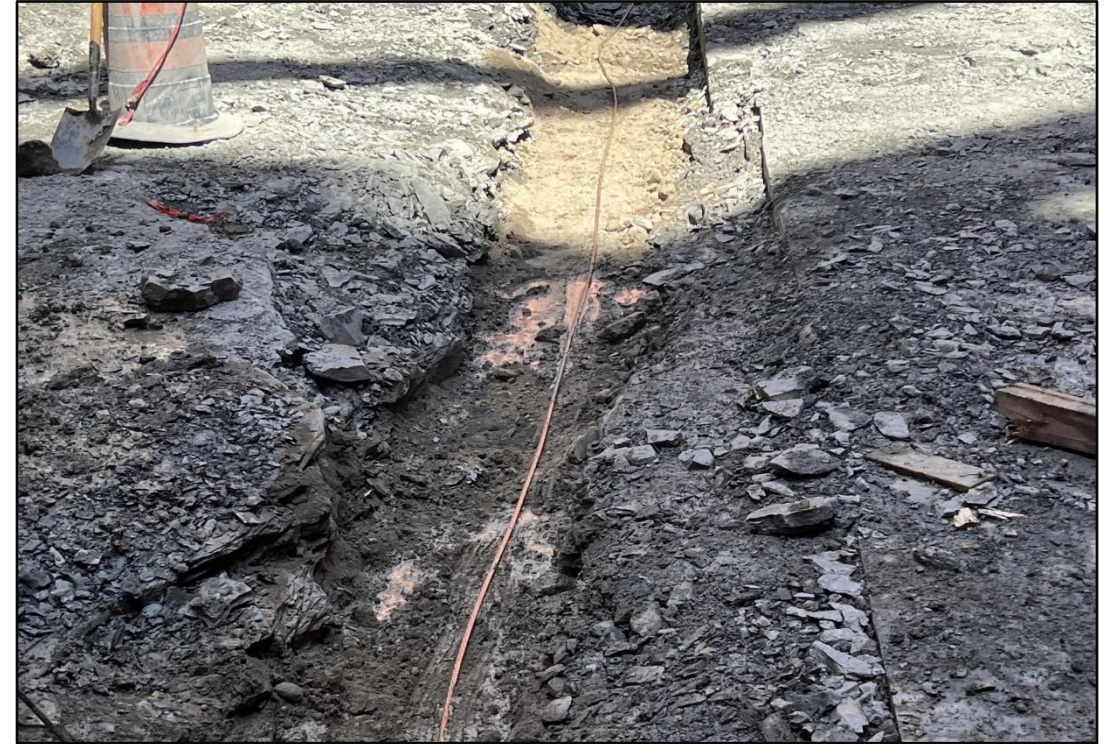
Trench dug with grounding cable in position
