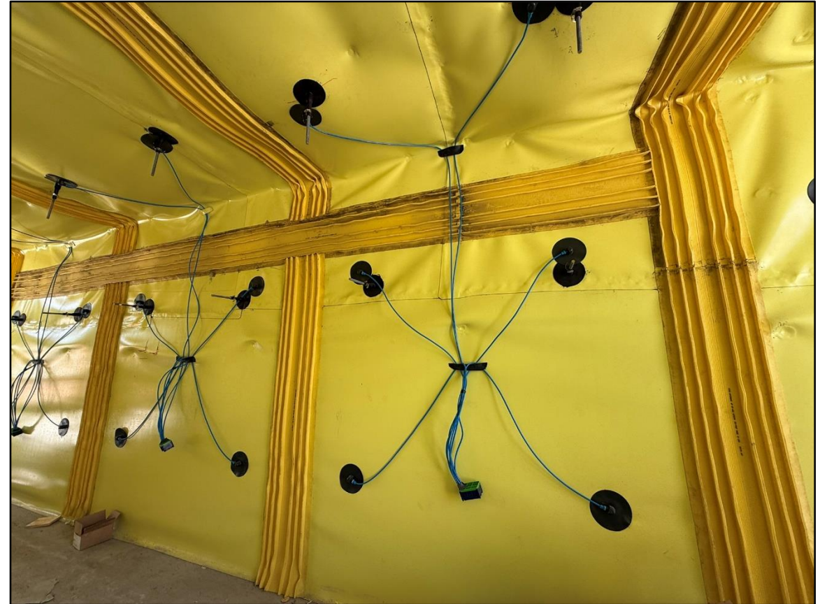
Waterproofing system testing at site
