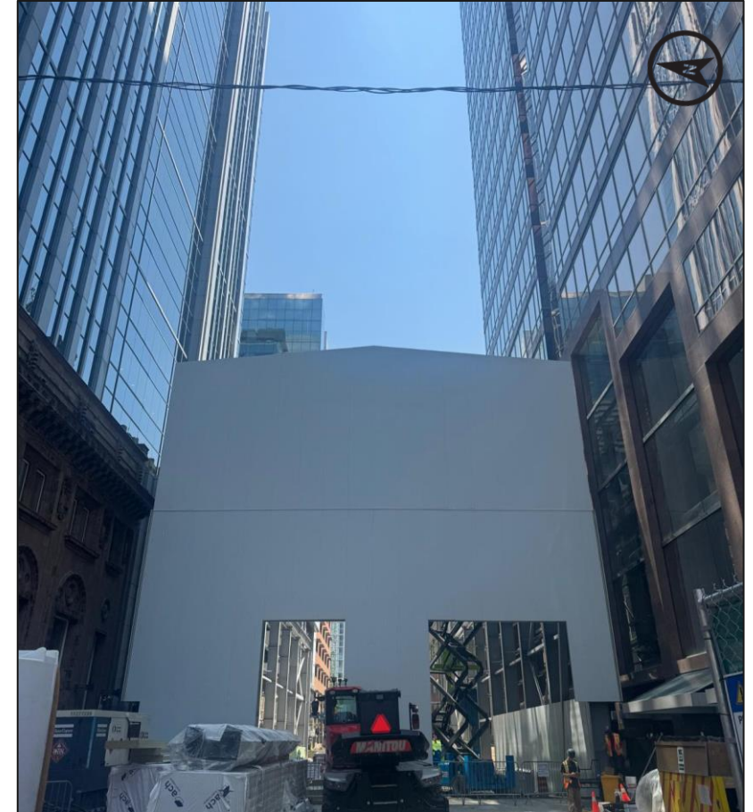
Cladding installation is underway for the future acoustic shelter at the Queen station east site.
