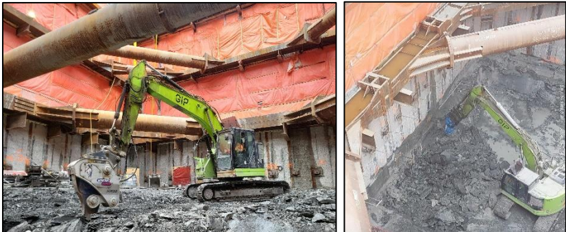
Noise blankets in use on large hammer attachment
