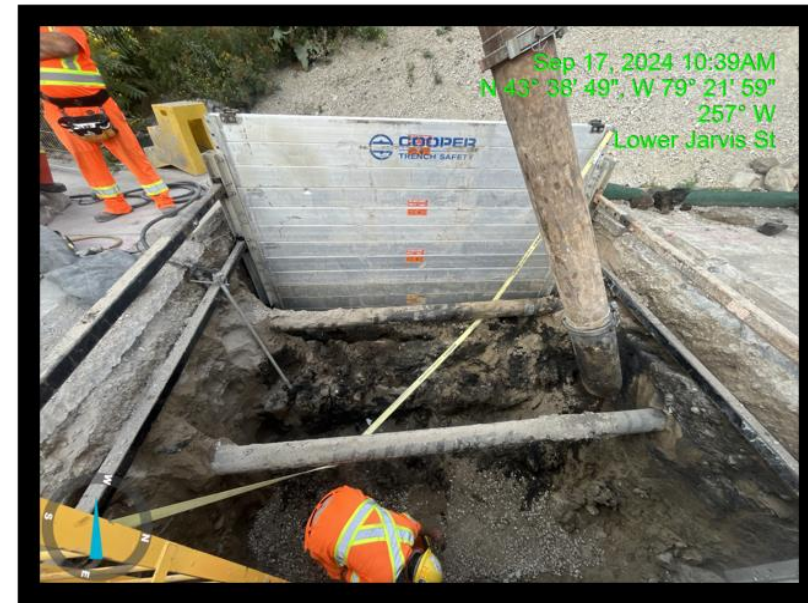
Wood timber uncovered during hydro-vac excavation at Lower Sherbourne Street West
