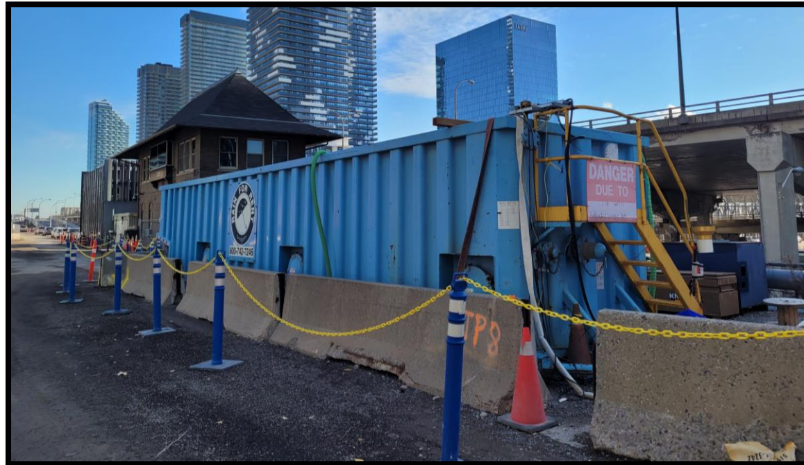
Construction dewatering holding tank, located near the Scott Street Tower
