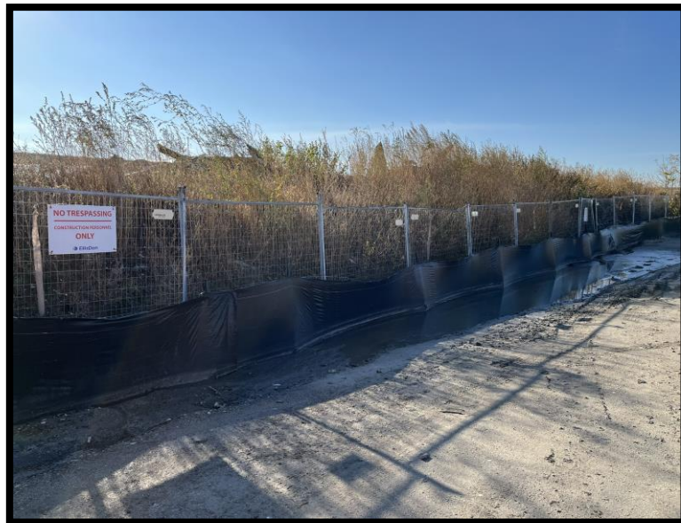
Silt fencing installed at Wilson Yard to prevent soil from migrating off-site
