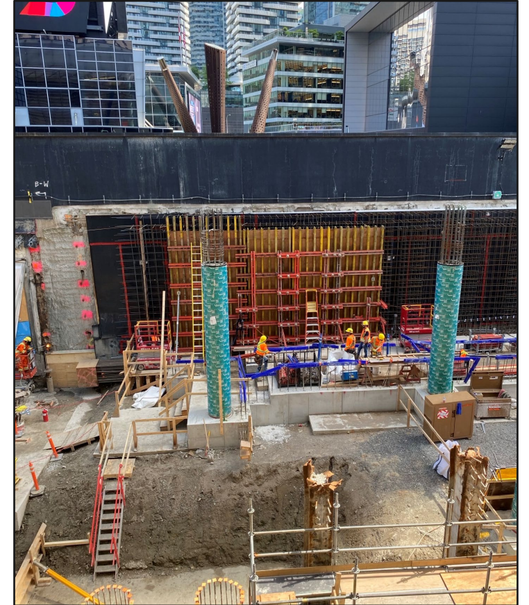
Photo: Area F/G - South wall formwork
