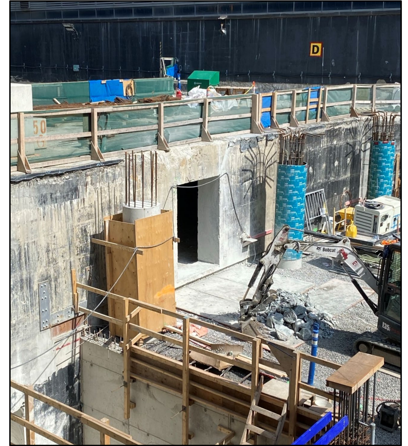
Photo: Truck Tunnel opening cut on the west side opening into Area C
