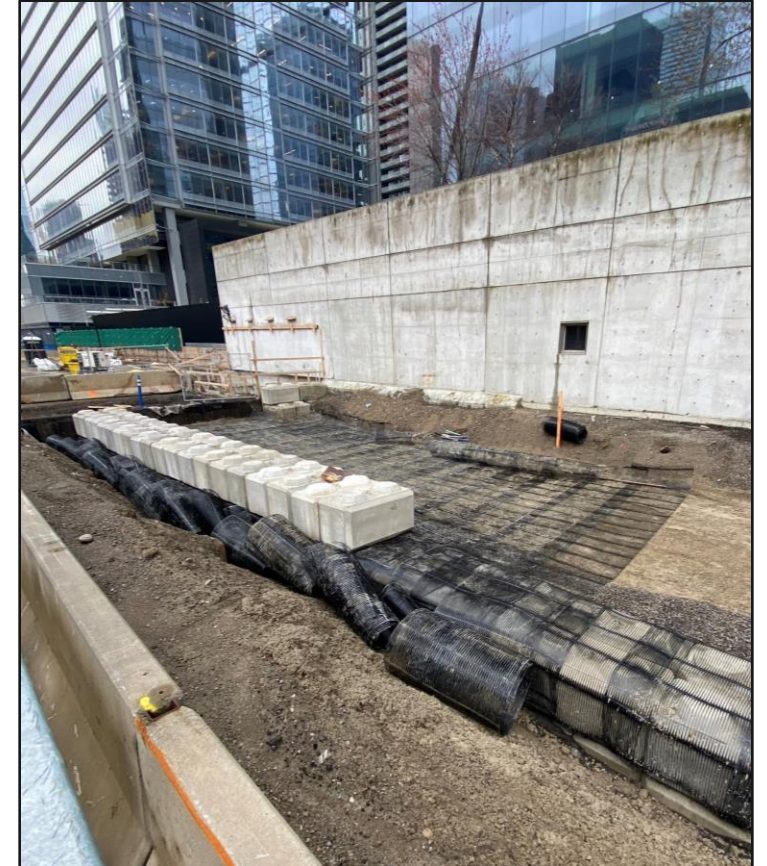
Photo: Lock block wall installations
