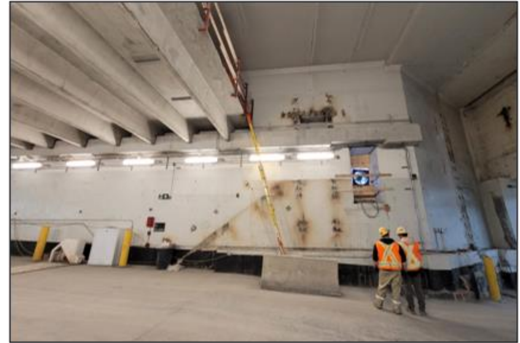
Photo: Truck Tunnel final Double Tee installation – before and after
