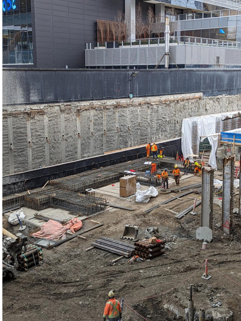
Photo: Area F/G Pile Cap Installation (Left image) and columns
