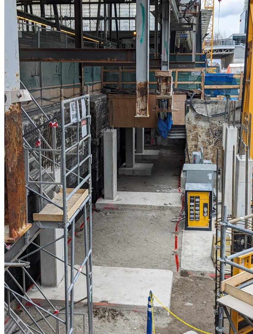
Photo: Area F/G Pile Cap Installation (Left image) and columns
