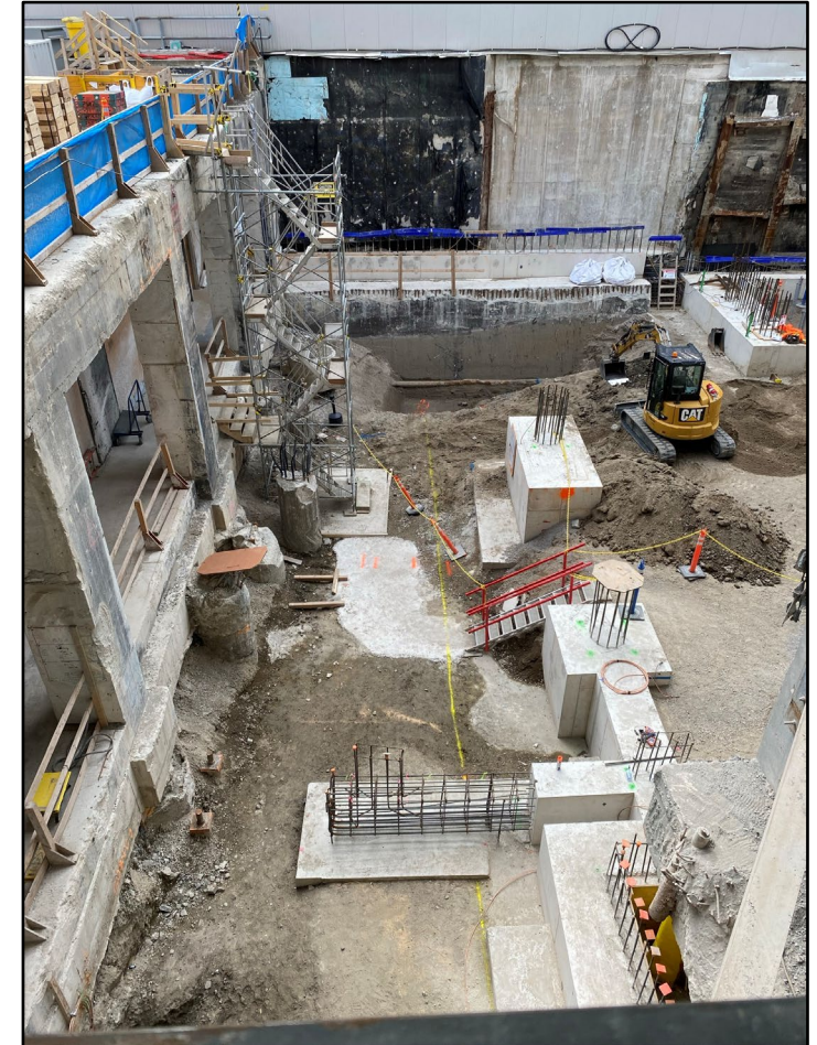
Photo: Area F/G - Final pile cap installation ongoing
