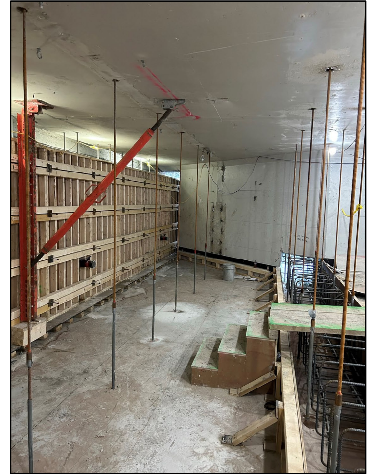
Photo: North beam formwork in OTA workspace above the truck tunnel
