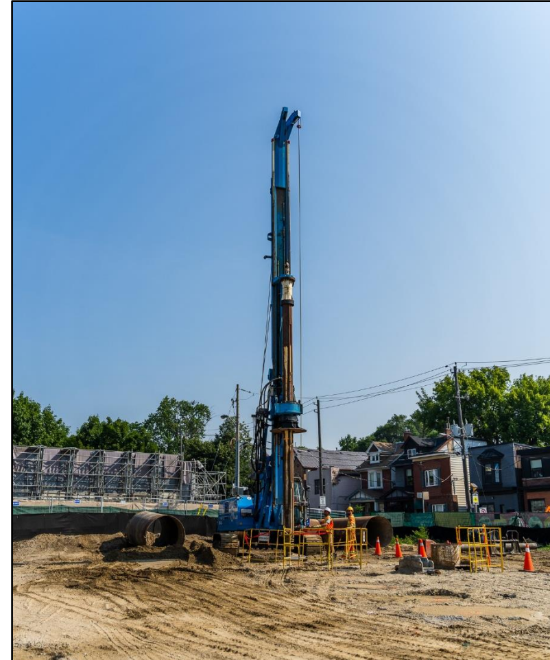
A drill rig performing piling works at the northeast end of the Gerrard Portal site.
