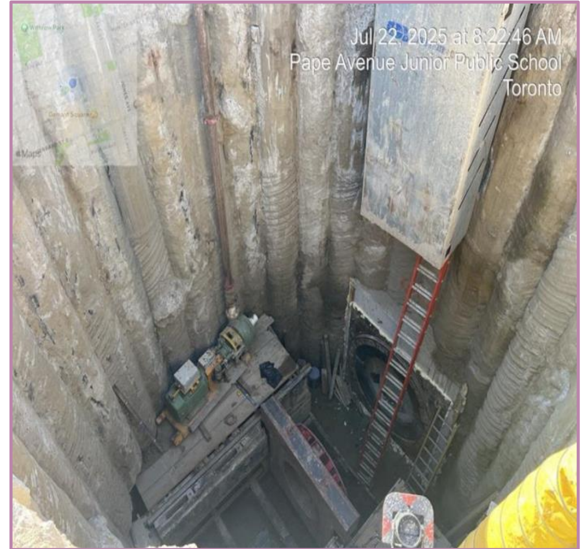
Microtunnel launch shaft - Riverdale
