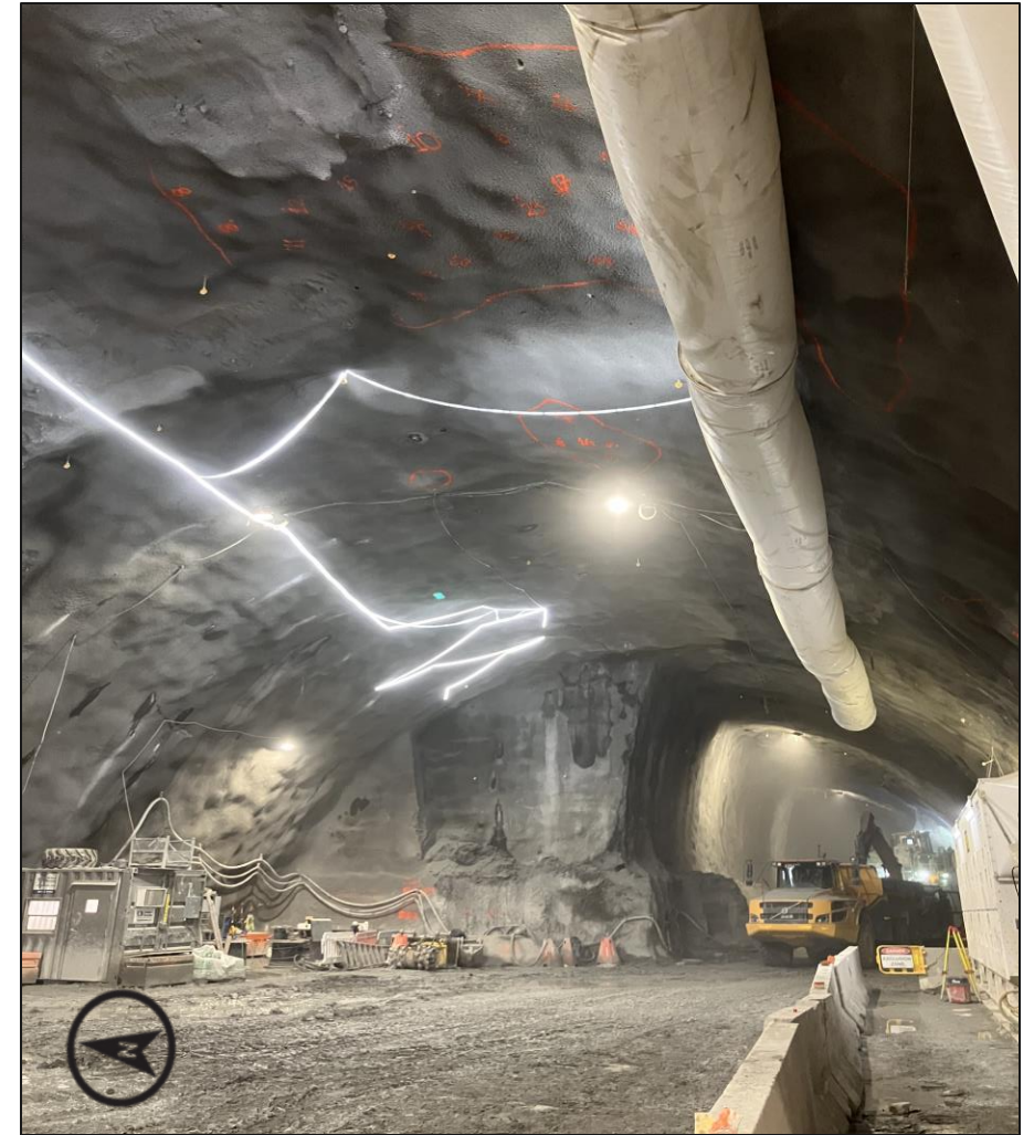
Machinery in the cavern at the Queen-Spadina station north site.
