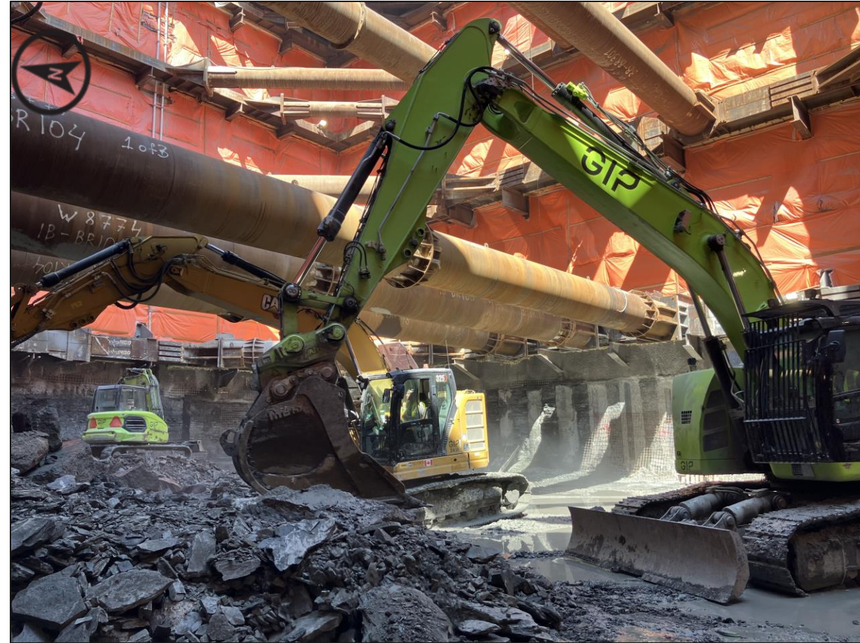
Excavation in progress at the Queen-Spadina south station site
