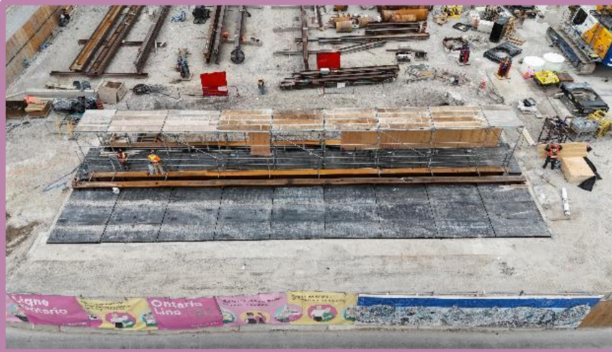
Covered bike lane overtop bridge decking, including overhead protection, in preparation for traffic shift
