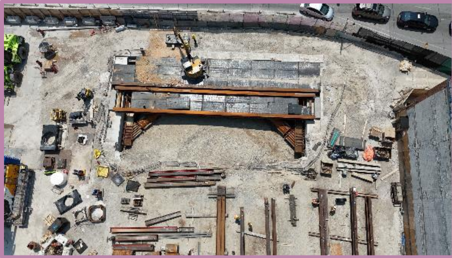
Overhead view of traffic decking
