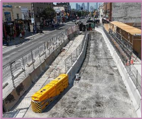
Asphalt new west bound lane, line painting and arrange traffic control barrier for new traffic control setup
