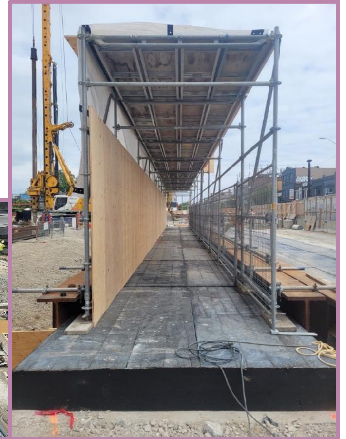
Covered bike lane overtop bridge decking, including overhead protection, in preparation for traffic shift
