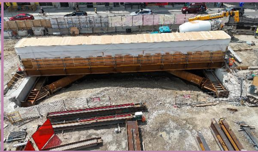
Covered bike lane overtop bridge decking, including overhead protection, in preparation for traffic shift
