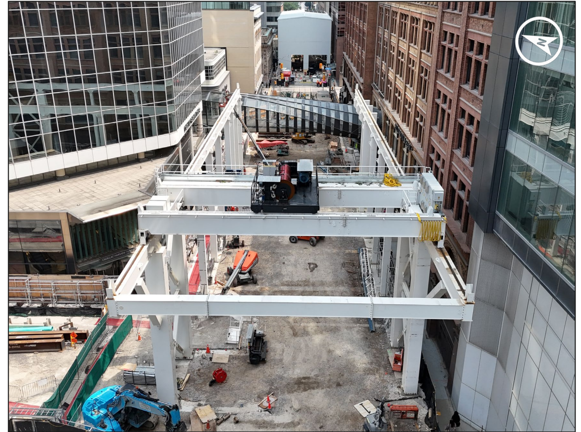
Example of gantry crane at Queen Station, similar crane to be installed on the east end of the portal.
