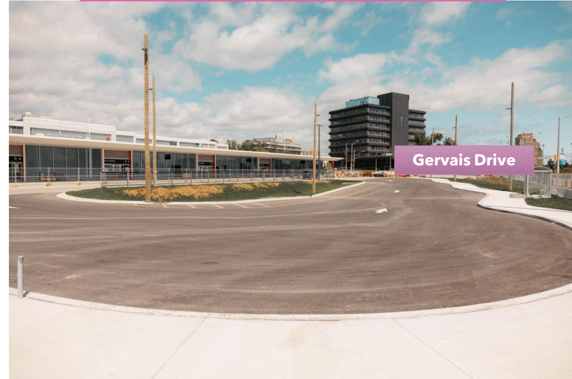
Temporary bus loop construction - view looking east
