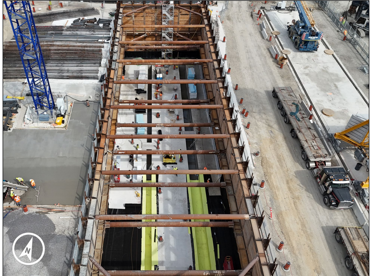
A view of permanent works at the future north entrance
