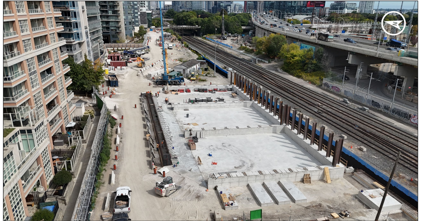
View of the preparation activities for future tunnelling.
