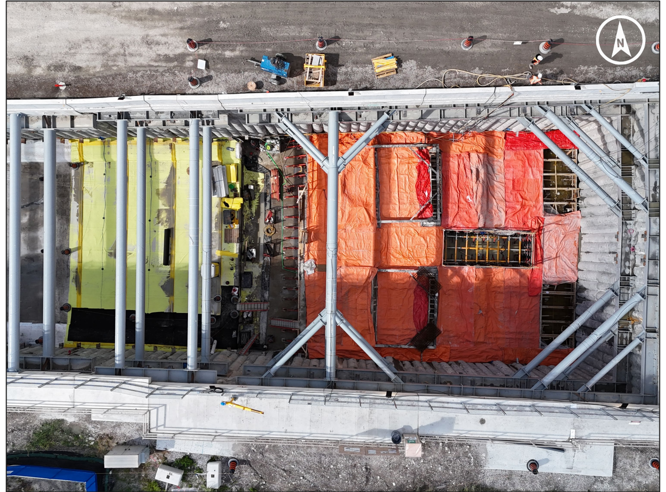
Aerial view of the permanent works at the portal
