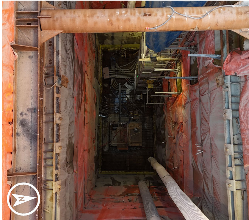
Aerial view down the shaft of the future EEB
