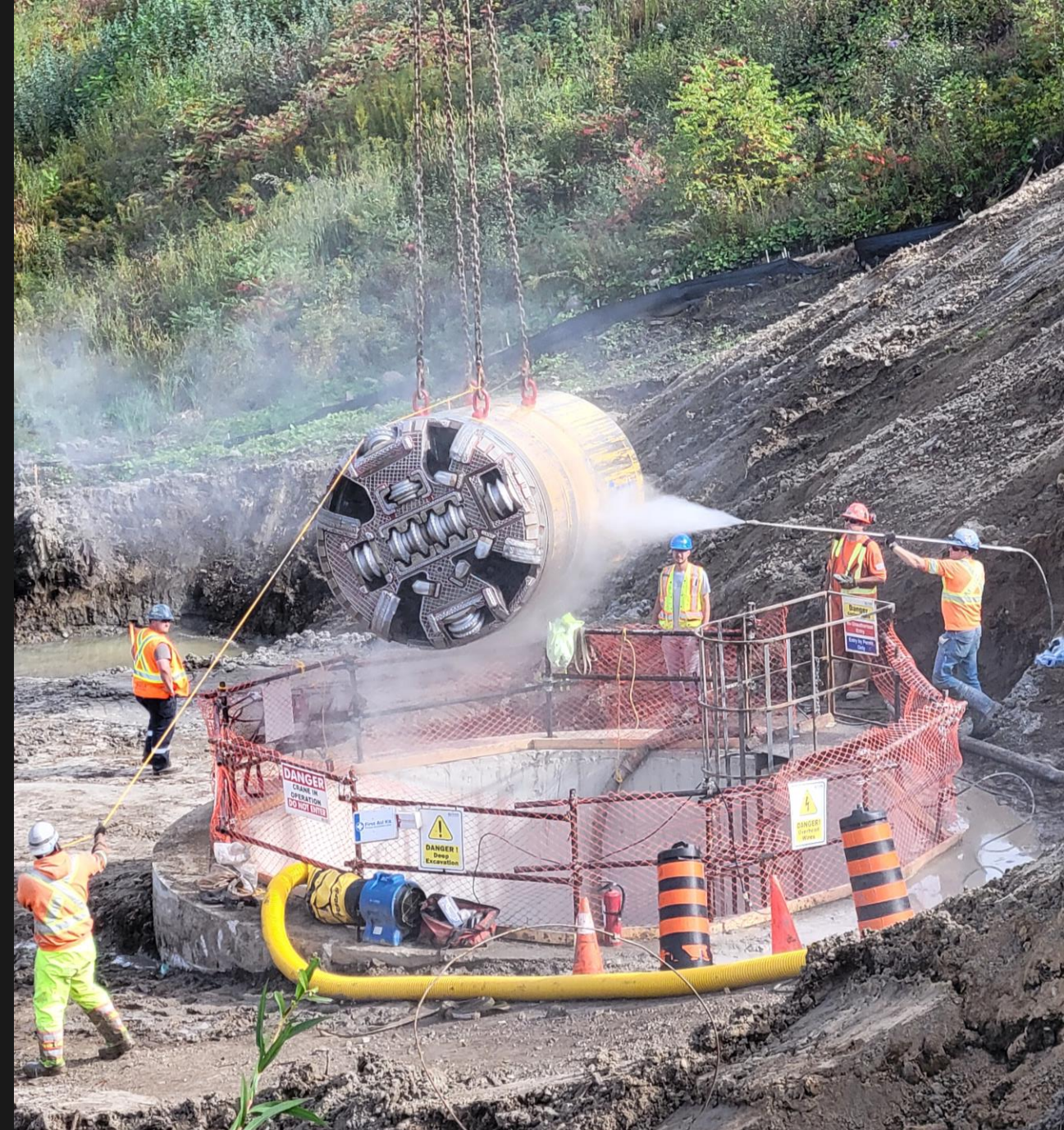
Tunnel boring machine used to dig new culvert
