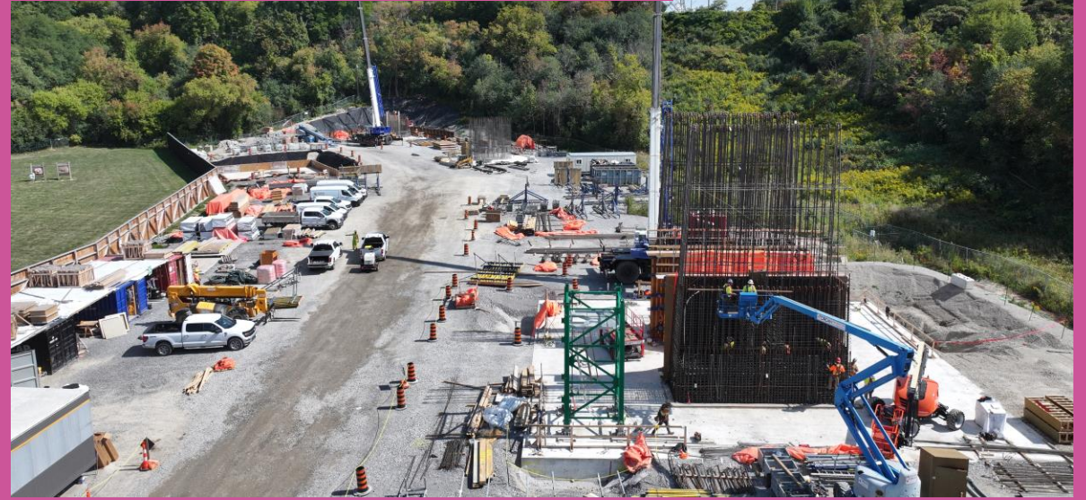
Future pier for the West Don bridge - September 2025
