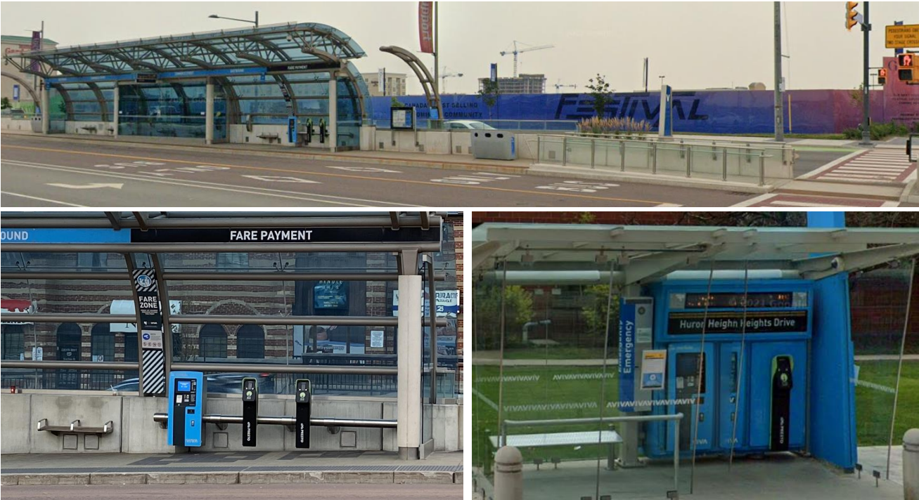
Figure 47: YRT VIVA Side Platform Stop (Top), Fare Payment Area Close-up (Bottom-left), and Bus Shelter (Bottom-right).
