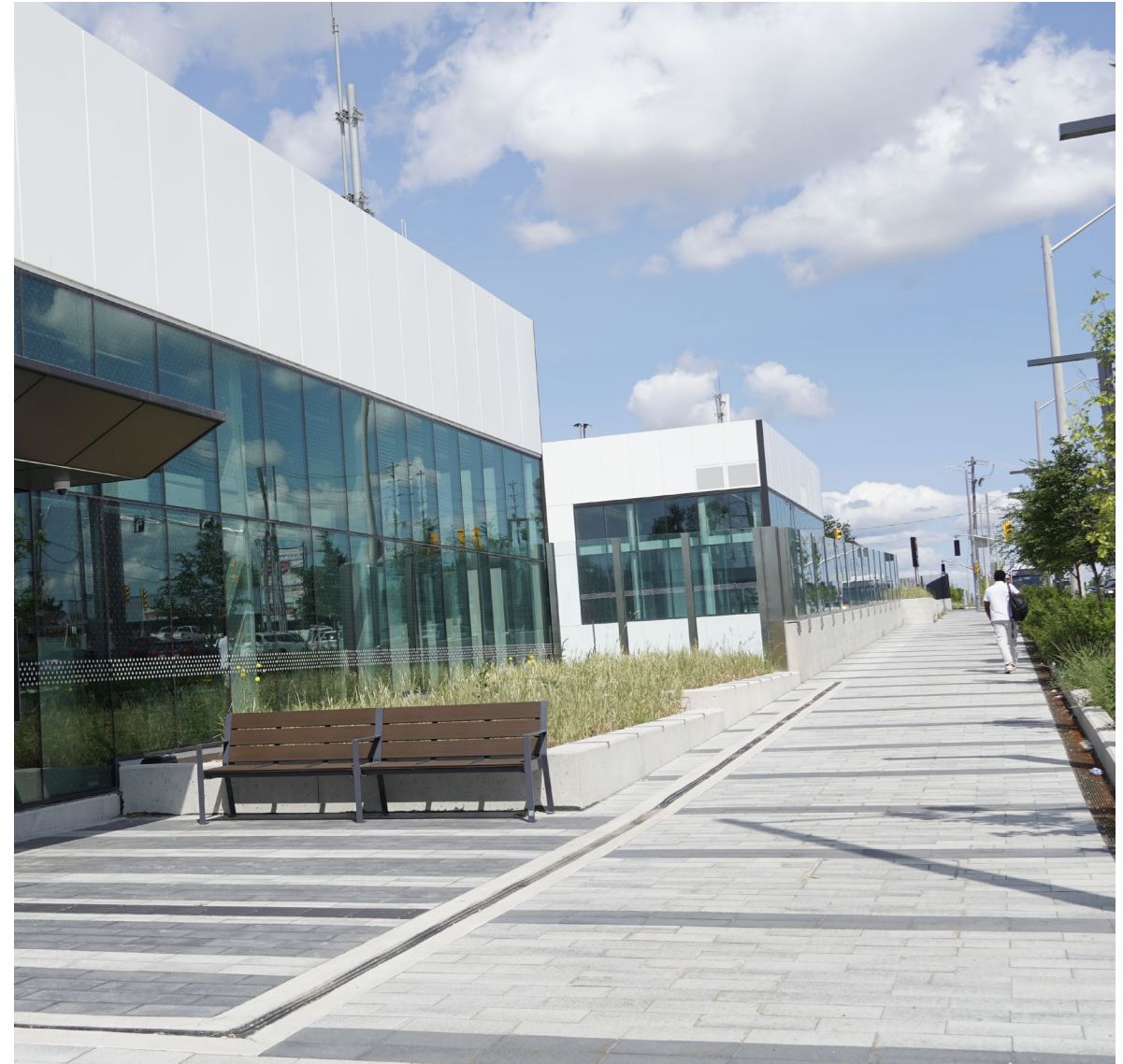
Photo: Humber College station walkway, view north. 2025.08.01
