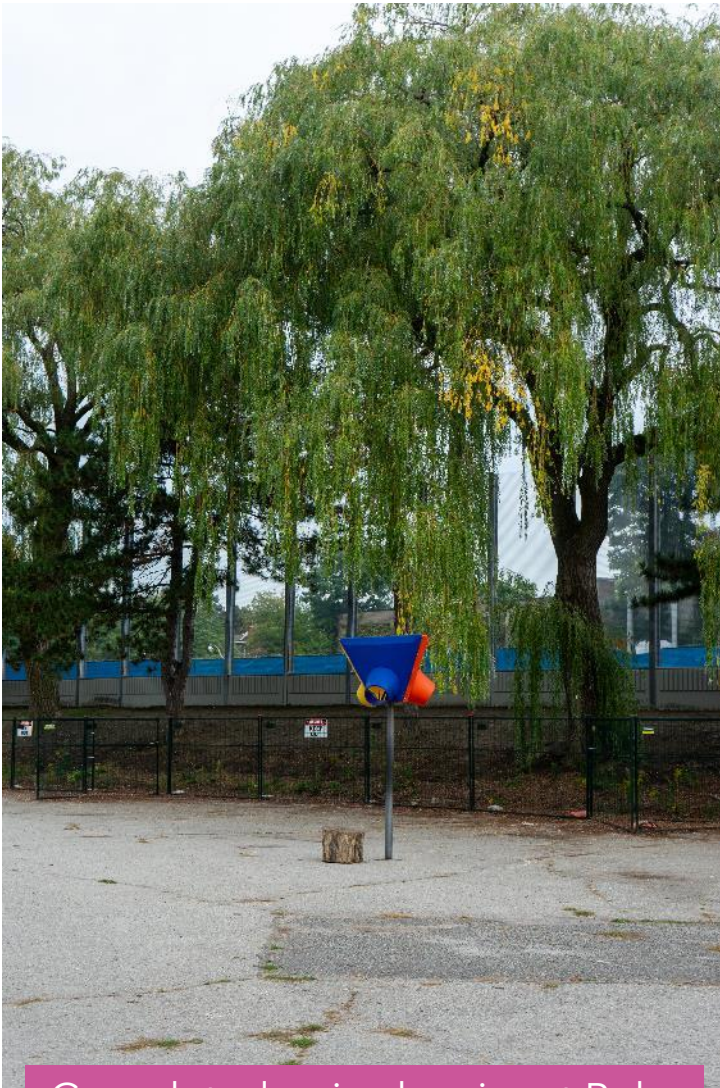
Completed noise barrier at Bake Jr. Public School - Sept. 24
