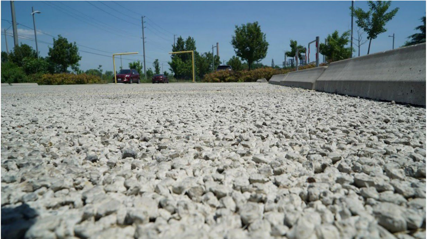
Figure 8: Permeable Concrete Paving at Lakeside Park, Mississauga
