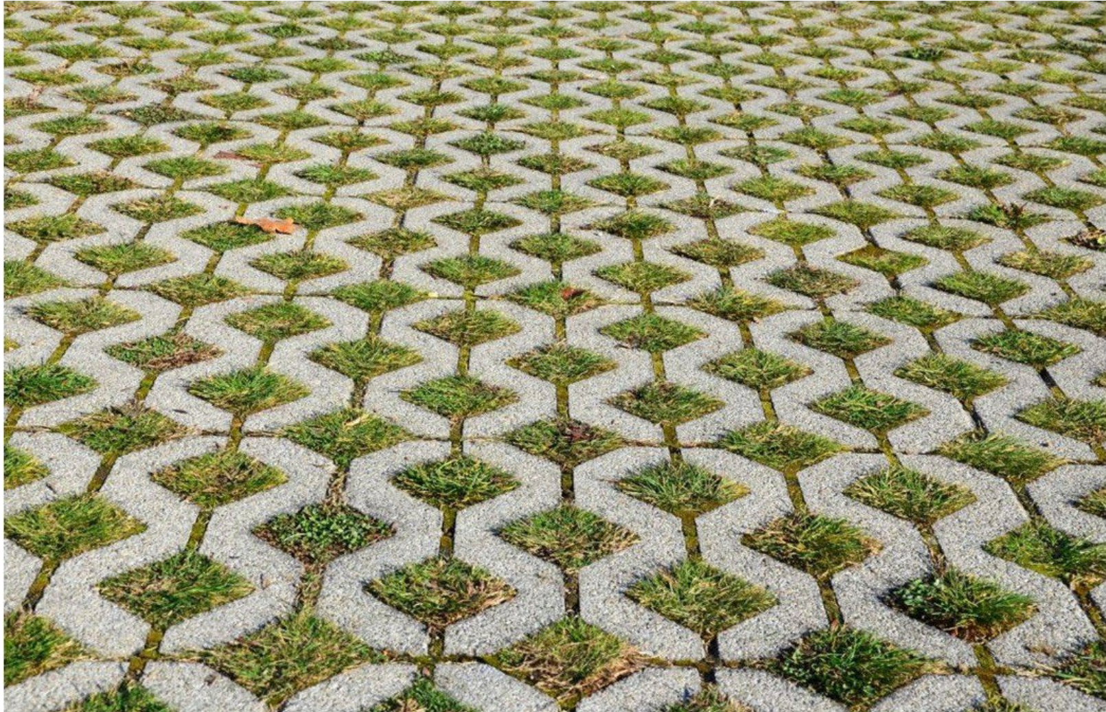
Figure 7: Concrete Open Grid
