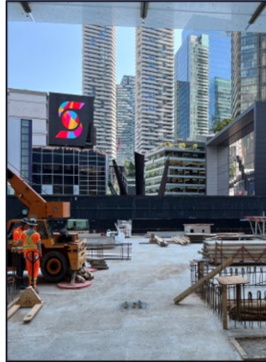
Photo: Track Slab Poured, September 2025
