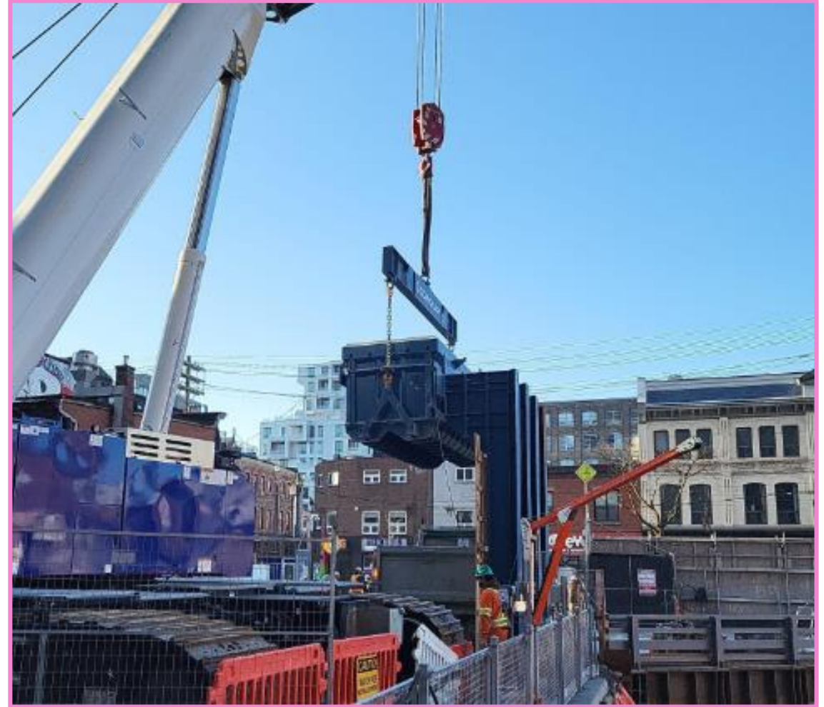
A self-dumping bin loading up a dump truck with excavated materials.
