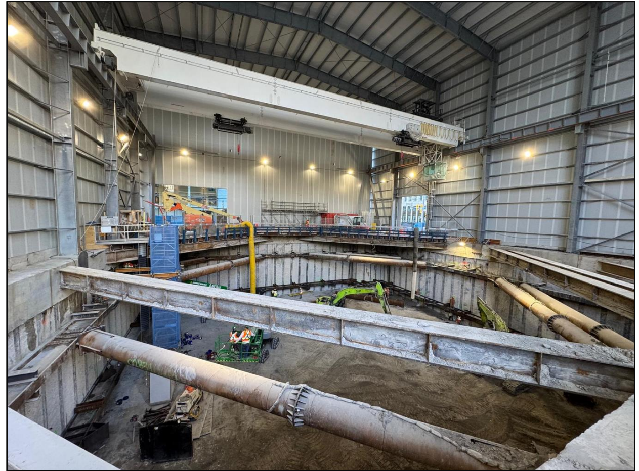
Shaft excavation inside the north acoustic shelter
