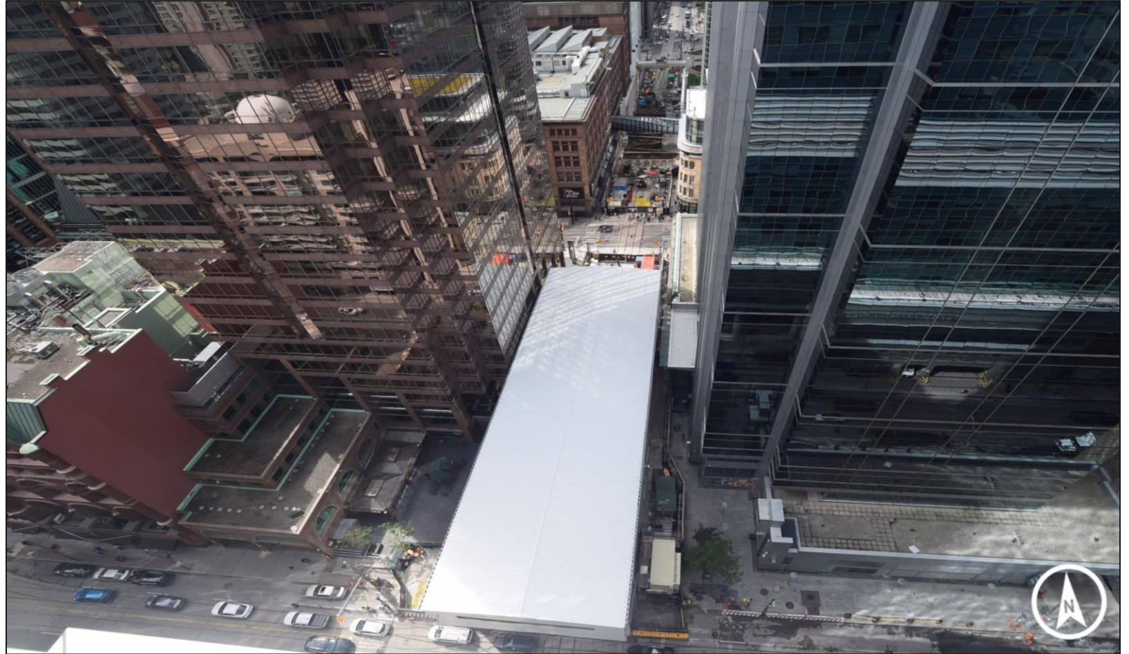
Aerial view of the acoustic shelter on the east site facing to the north direction
