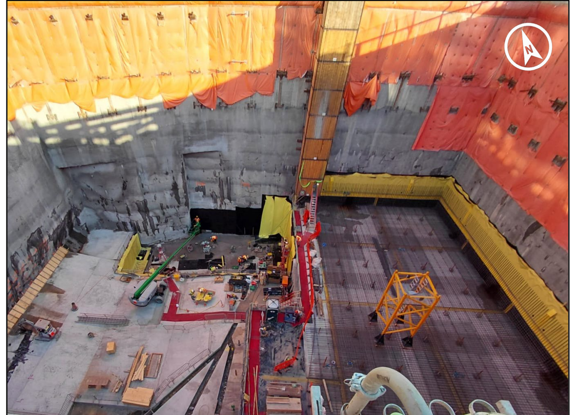
Mud slab, waterproofing, rebar and the second tower crane installation
