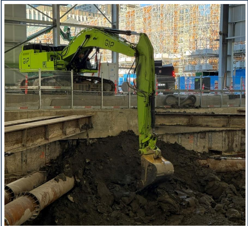
Soft soil excavation at the north end of the north shaft
