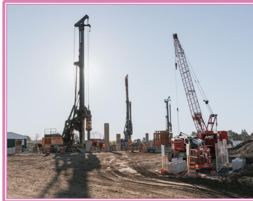
Launch Shaft Preparation
