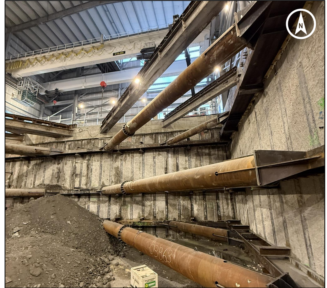
Three levels of strut and walers and gantry crane above
