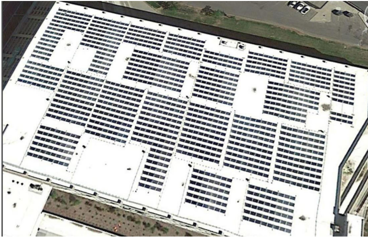
Erindale GO Station, 250 kW, Installed 2013
