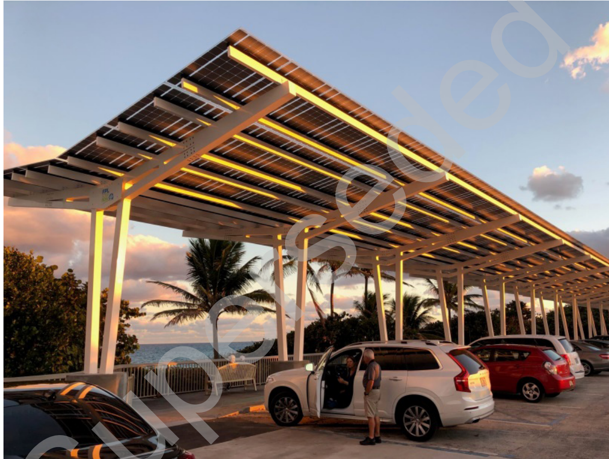
Solar Carport, Oceanfront Park, Boynton Beach, Florida (Source: lumossolar.com)
