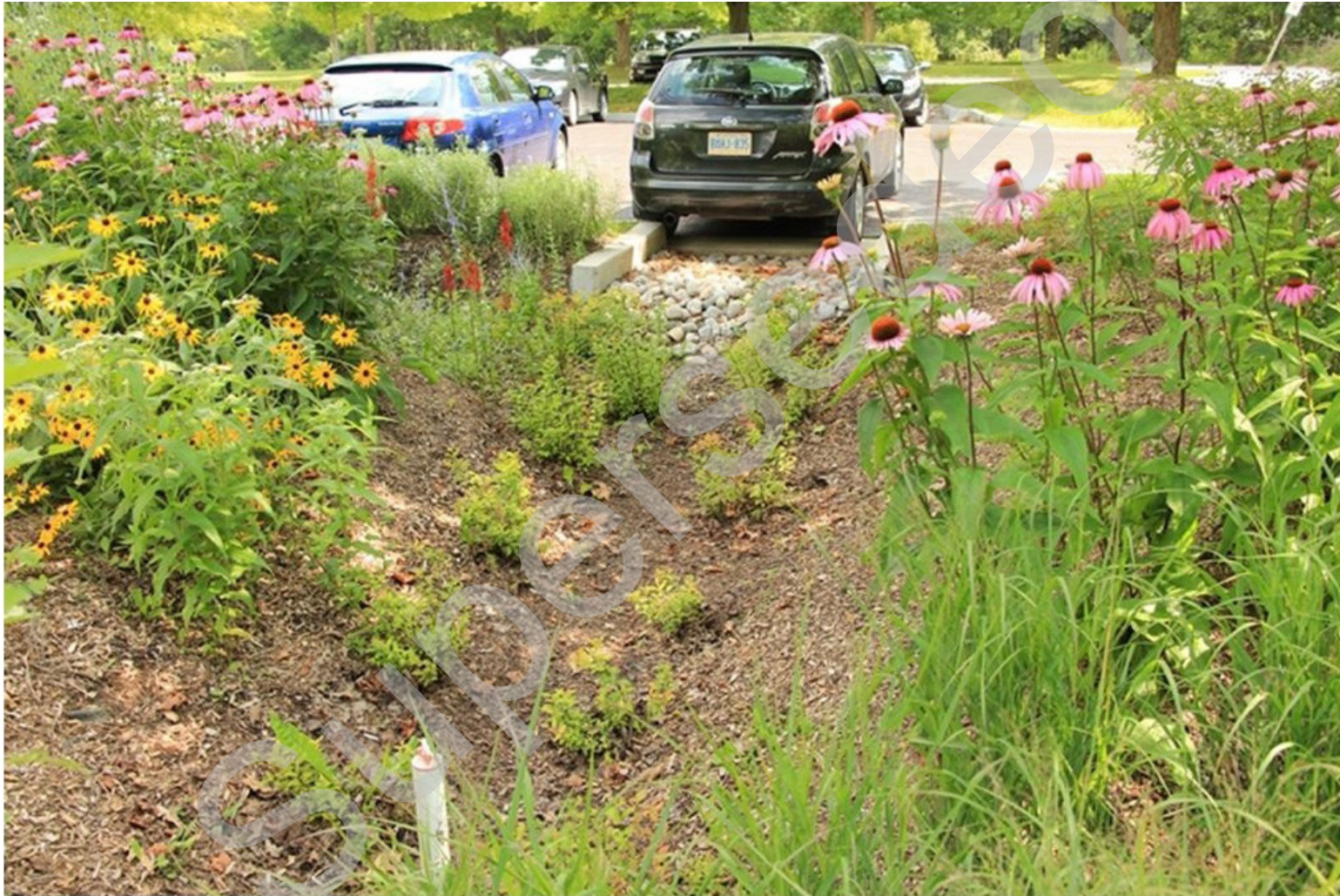
Bioretention Cell capturing and treating runoff from adjacent parking lot (Source: Sustainable Technologies)
