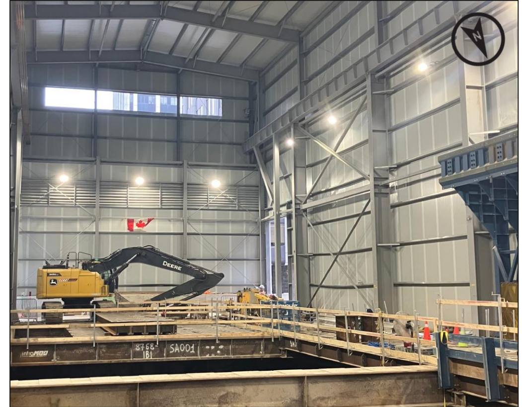
Excavation is underway inside the acoustic shelter at the Queen Station east site
