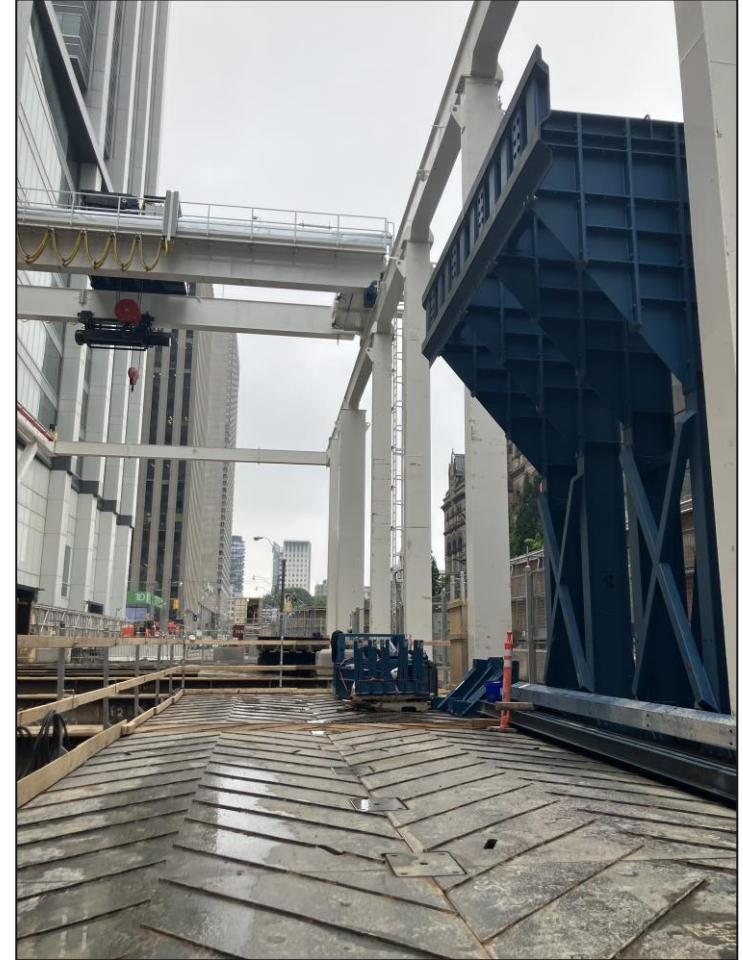
Deck installation at the Queen west site
