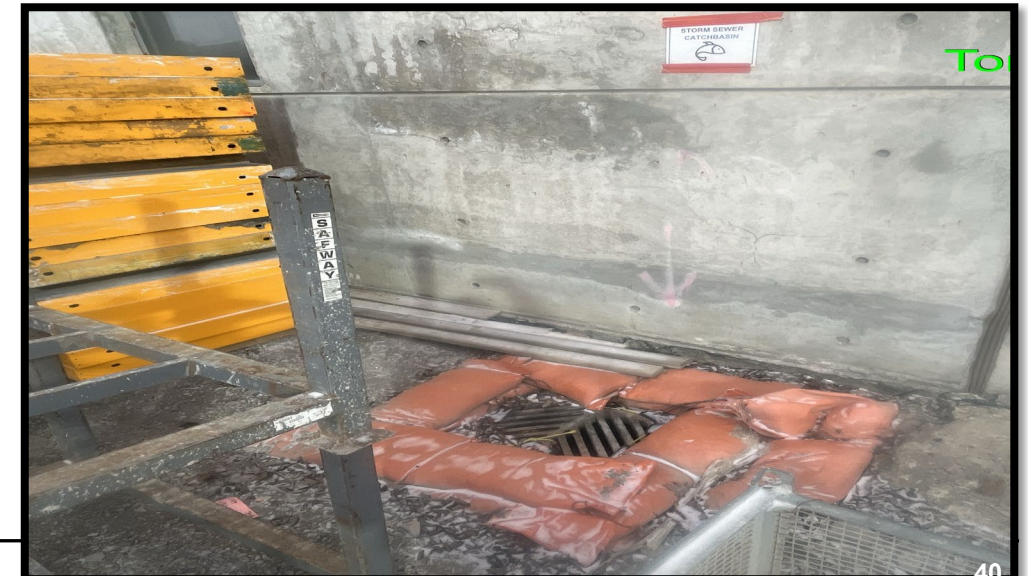
Catch Basin inlet with sandbag barrier
