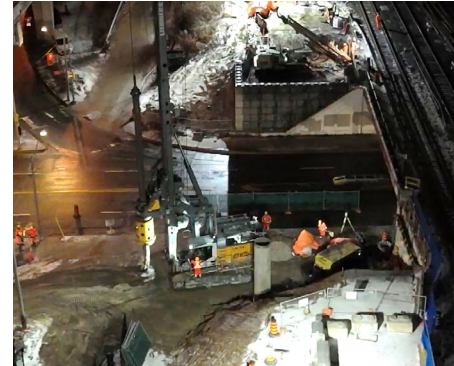
Installed new caissons foundation
