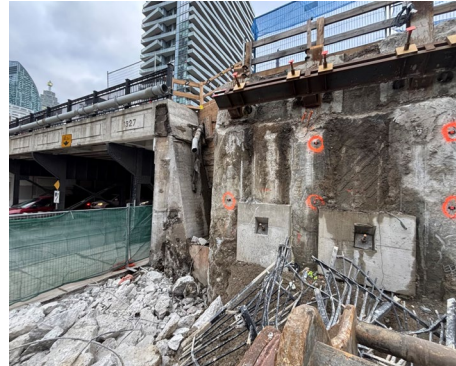
Demolished old wingwall and bridge fascia
