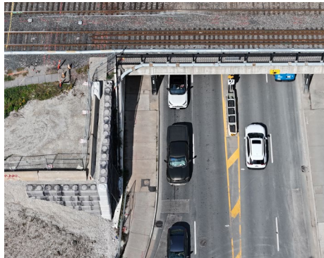
Installed secant wall
