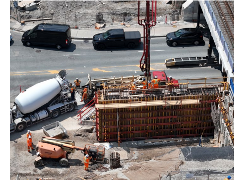
Poured concrete for new abutments at both bridge locations
