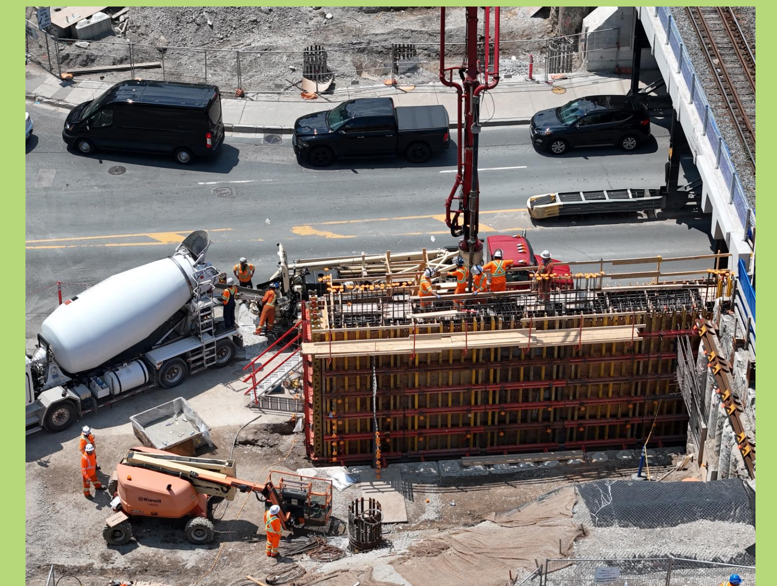
Poured concrete for new abutments at both bridge locations
