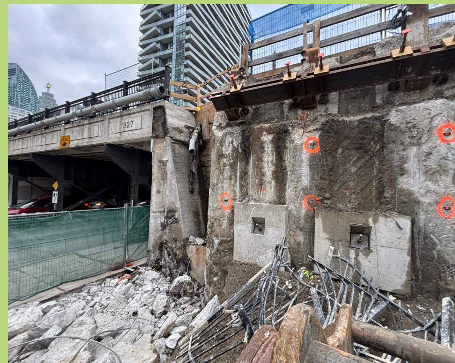
Demolished old wingwall and bridge fascia
