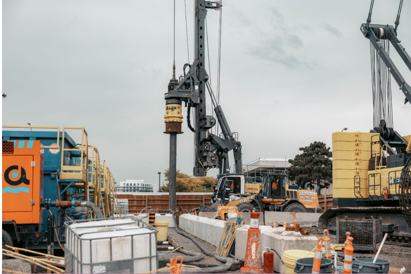
Drilling at D-41 - Oct 21, 2025
