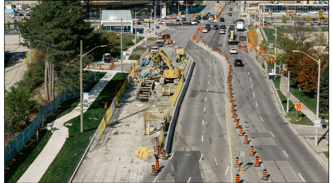
Northbound view on Don Mills Road at Eglinton Avenue East – November 2, 2025
