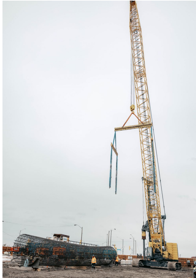
Rebar cage at D-40 - Oct. 21, 2025
