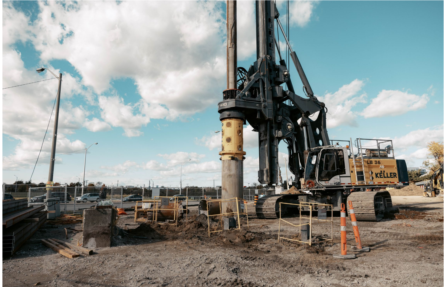
Support of excavation drilling just north of Wynford Drive
