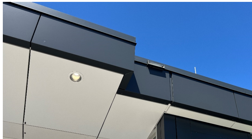
Figure 6.1: Metal Cap Flashing
