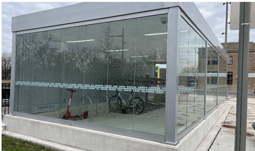
Figure 7.8: Exterior Glazing with Bird-Friendly Frit and Distraction Pattern
