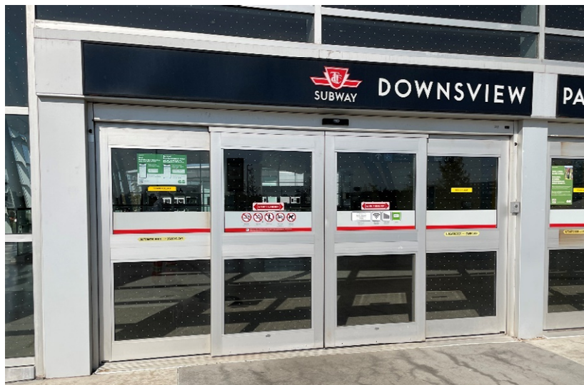
Figure 7.2: Aluminum Sliding Doors
