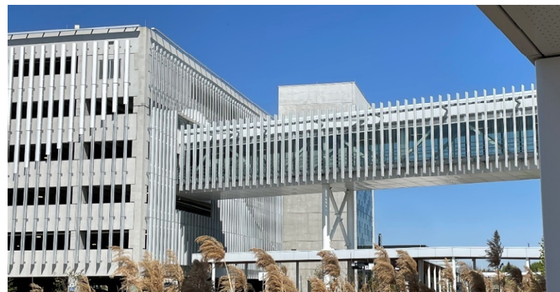
Figure 4.8: Exterior Aluminum Fins
