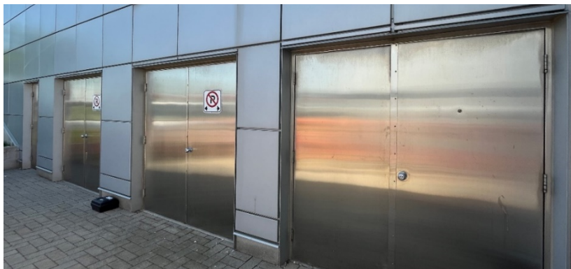
Figure 7.1.3: Stainless Steel Swing Doors
