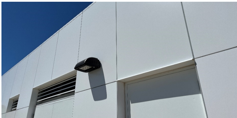
Figure 4.3: Prefinished Aluminum Panel Cladding
