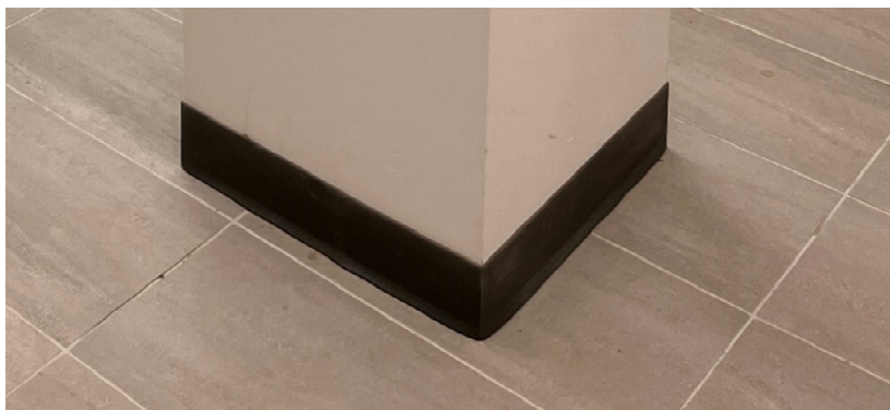
Figure 3.9.1: Non-integrated Rubber Wall Base
