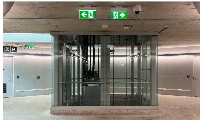
Figure 8.4: Glass Enclosure Around Elevator Shaft
