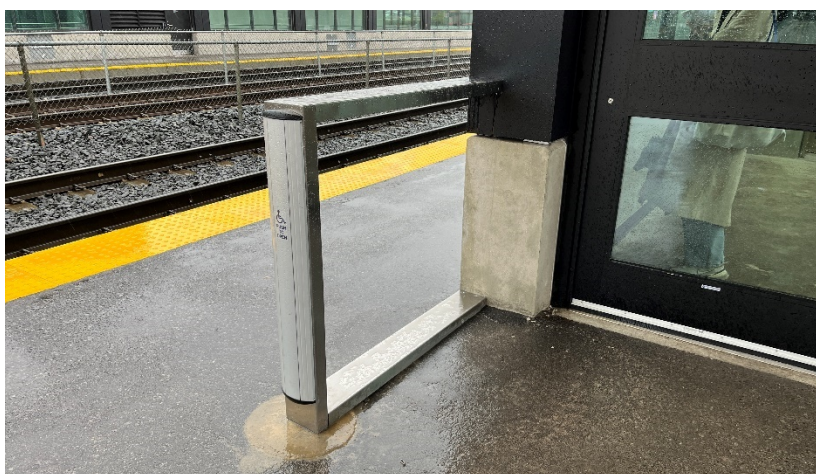
Figure 7.7.8: Automatic Door Operator
