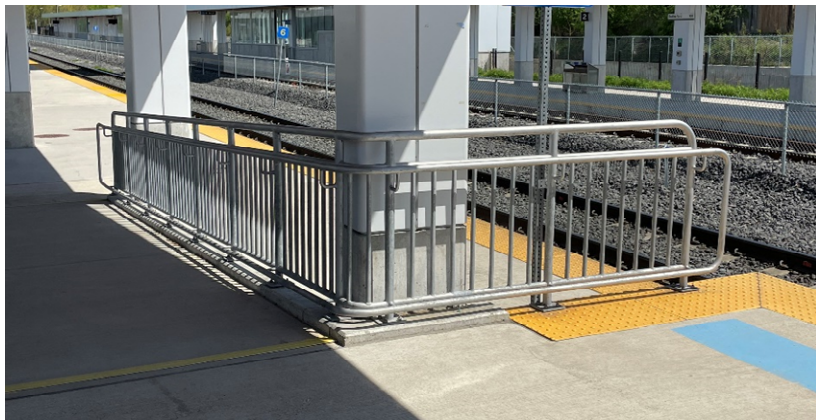
Figure 8.3: Galvanized Steel Guard and Handrail
