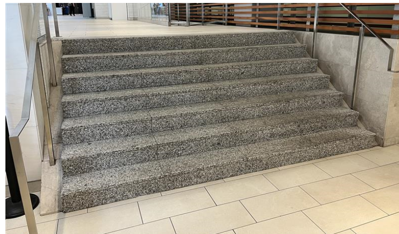
Figure 3.7: Granite Floor Finish at Stairs
