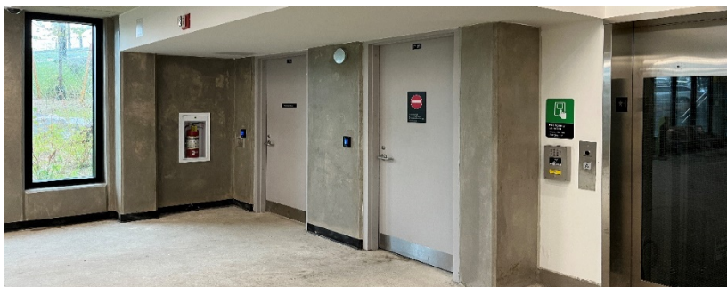
Figure 7.1.2: Hollow Metal Swing Door
