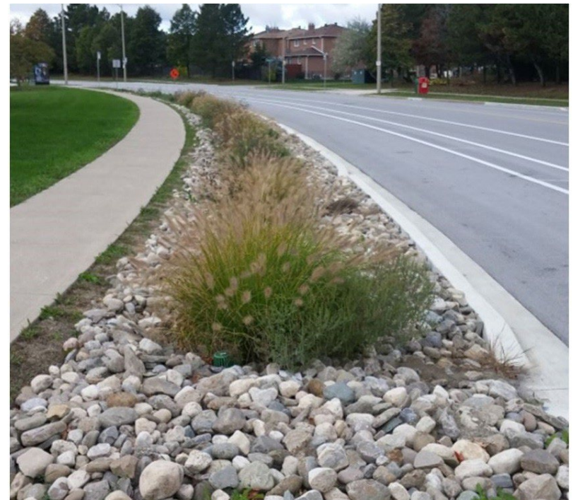
Figure 10: Bioswale along Country Code Court Boulevard in Brampton
