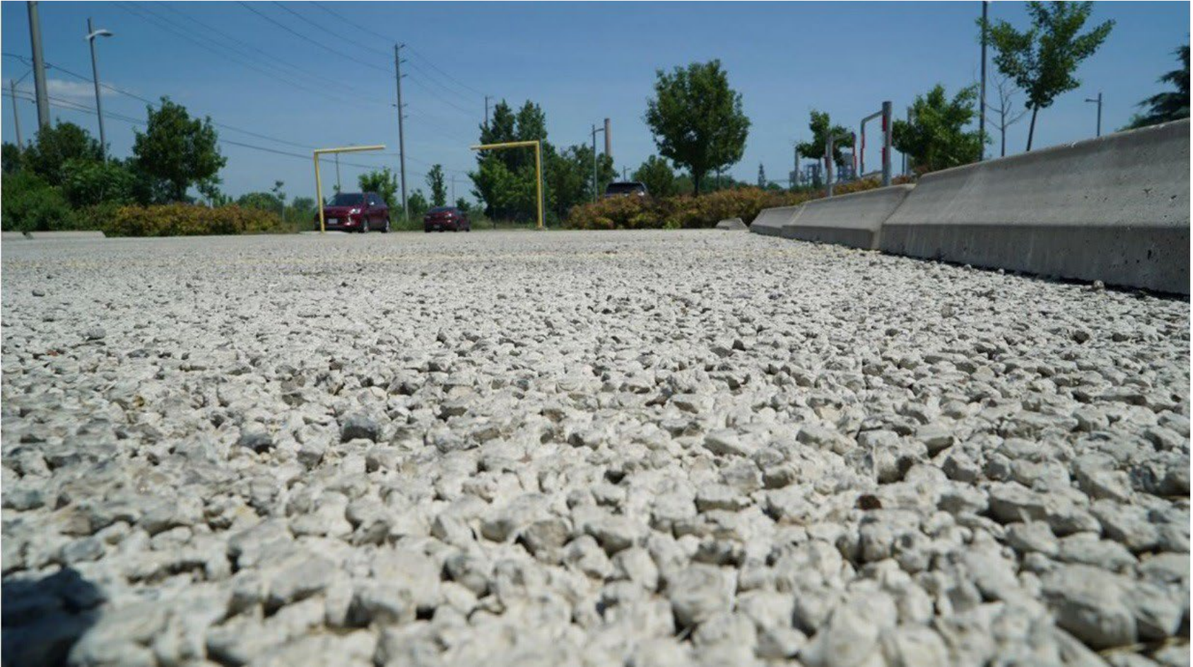
Figure 8: Permeable Concrete Paving at Lakeside Park, Mississauga
