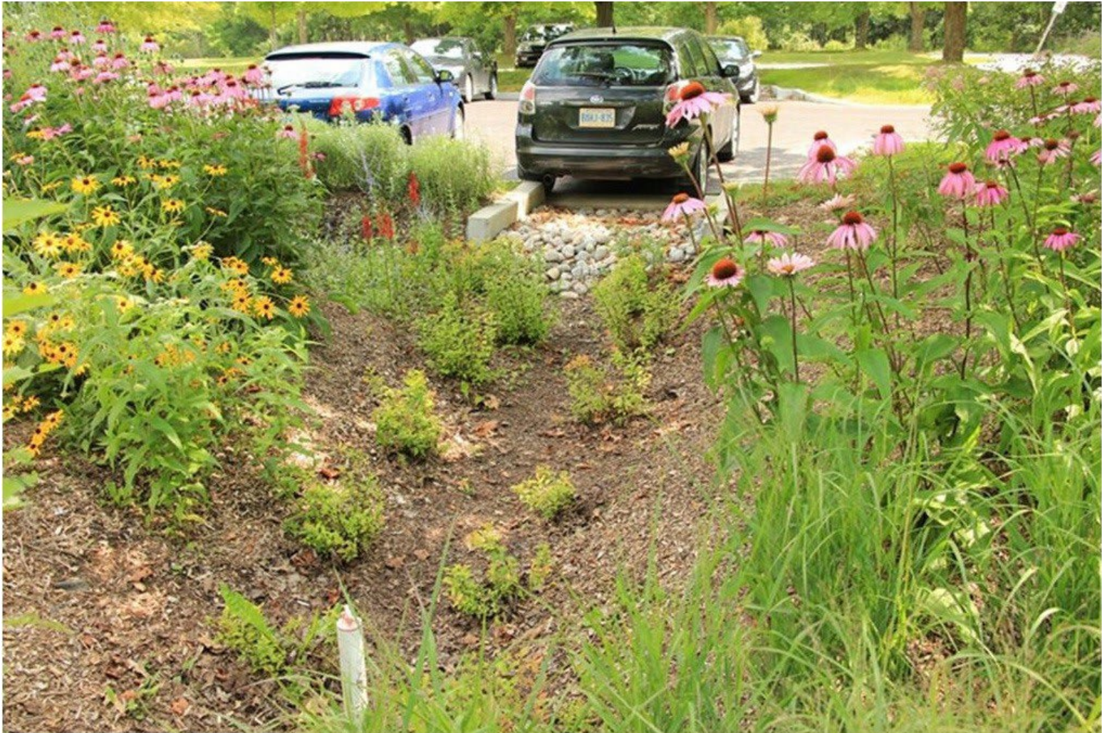
Figure 9: Bioretention Cell Capturing and Treating runoff from Adjacent Parking Lot
