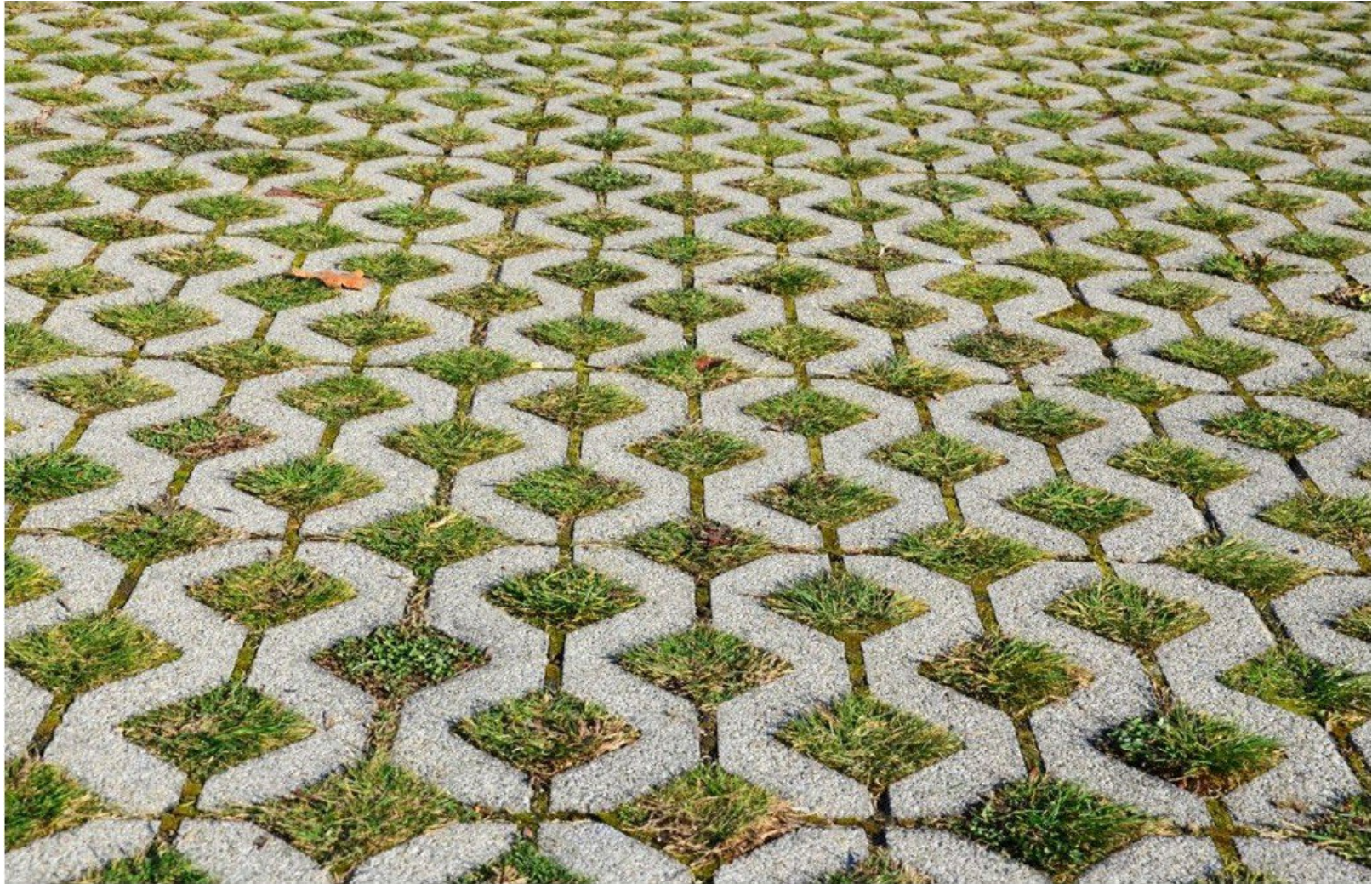
Figure 7: Concrete Open Grid
