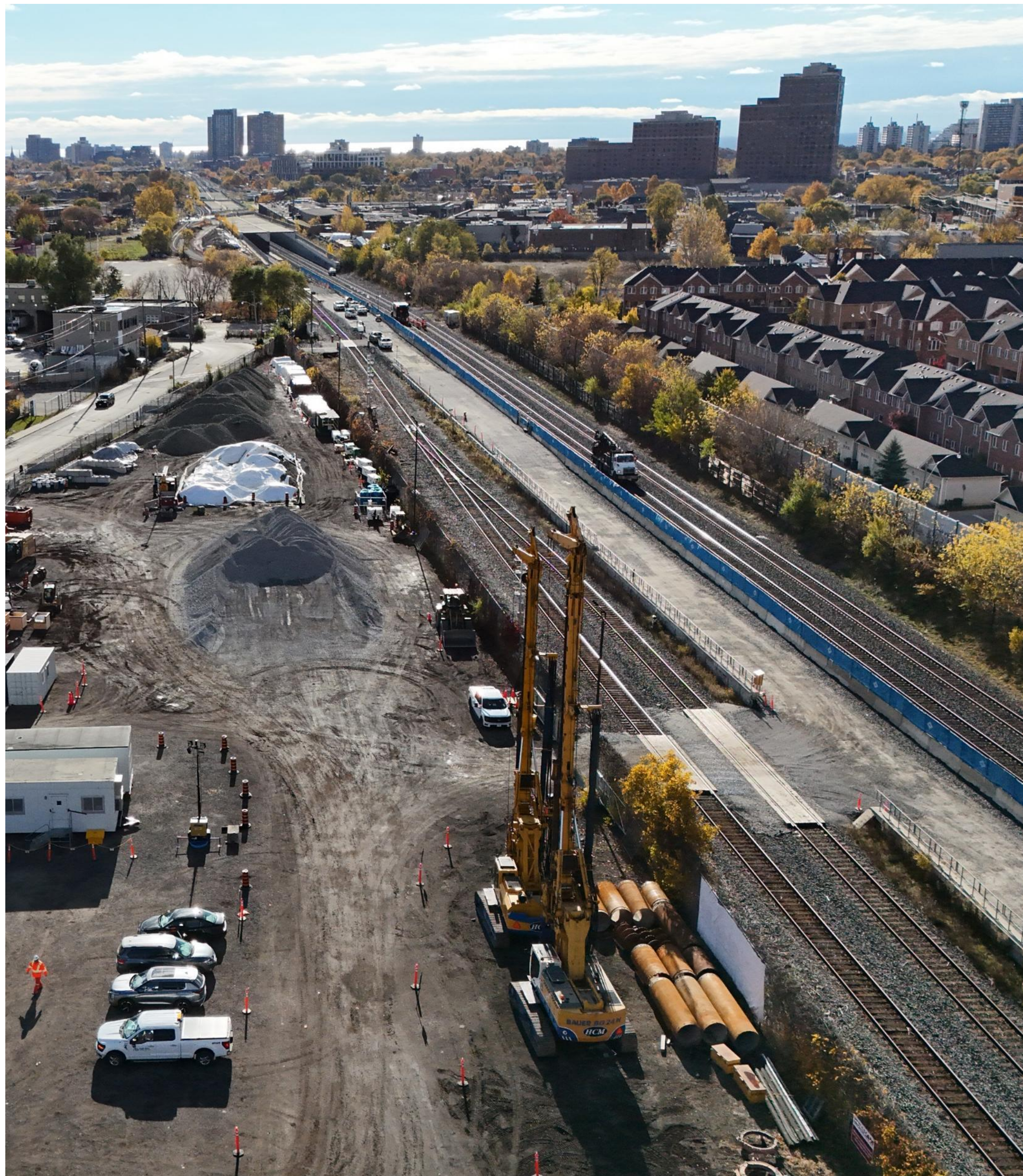
Site of the future station featuring the expanded Continuous Work Zone.
