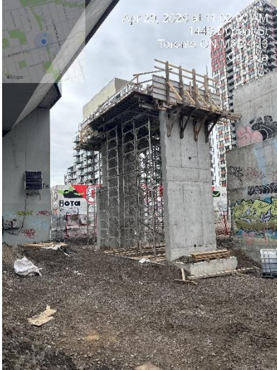
#2 Pedestrian Bridge abutment construction near Dupont St
