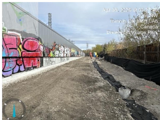
#1 In-corridor works near Davenport Village Park
