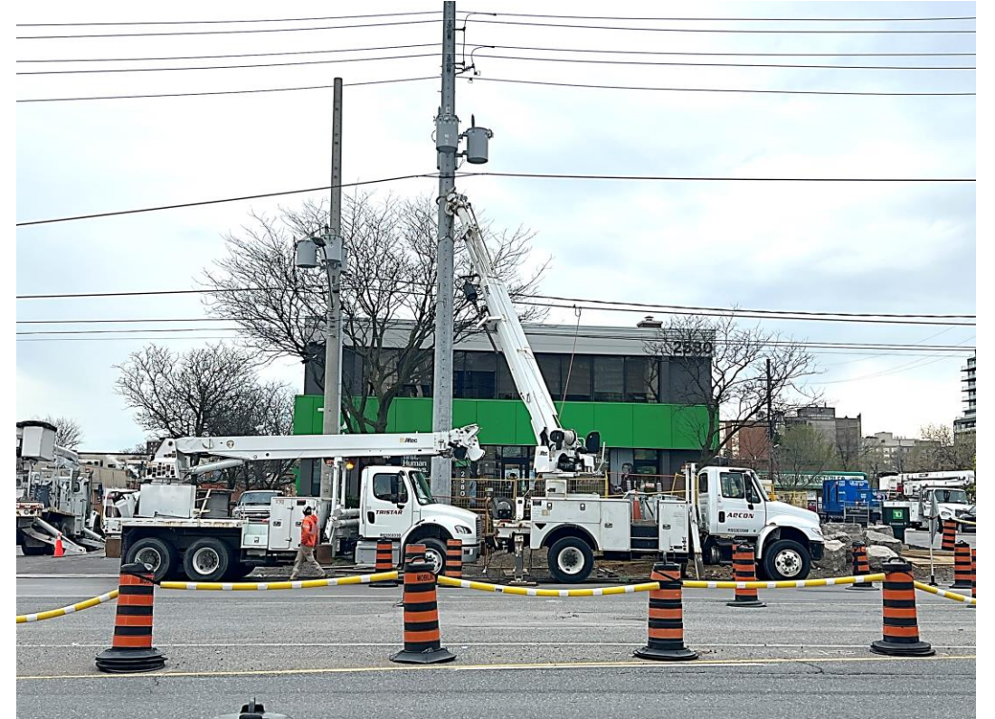
West side of Hurontario Street south of Dundas Street
