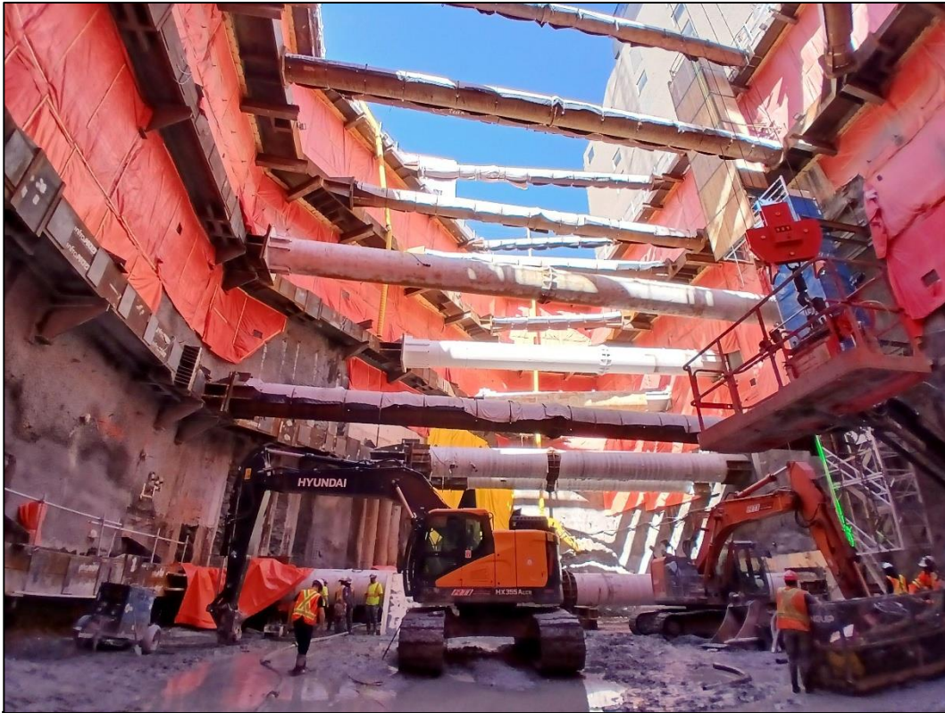
View from the south King West station site shaft facing north.
