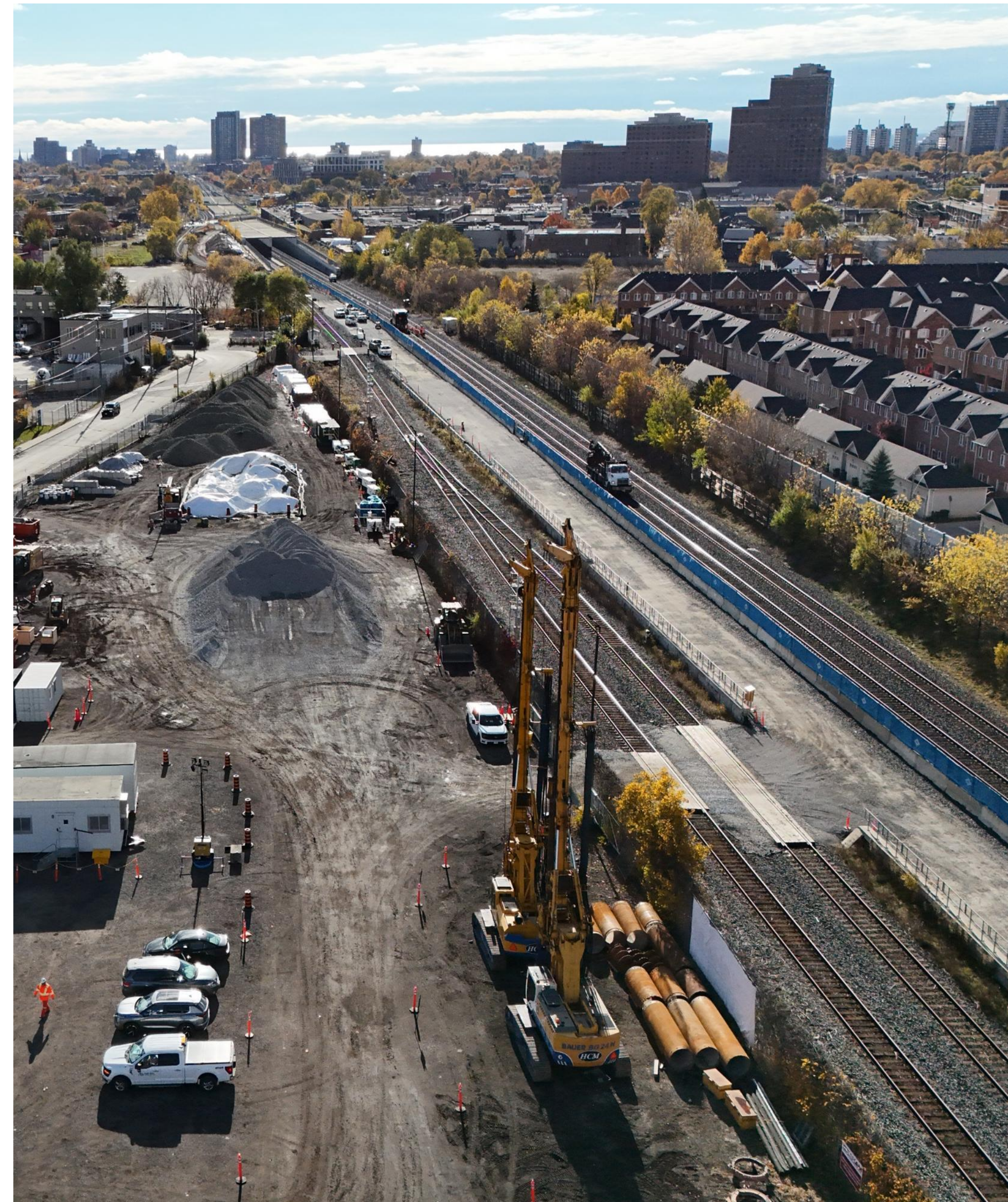
Site of the future station featuring the expanded Continuous Work Zone.
