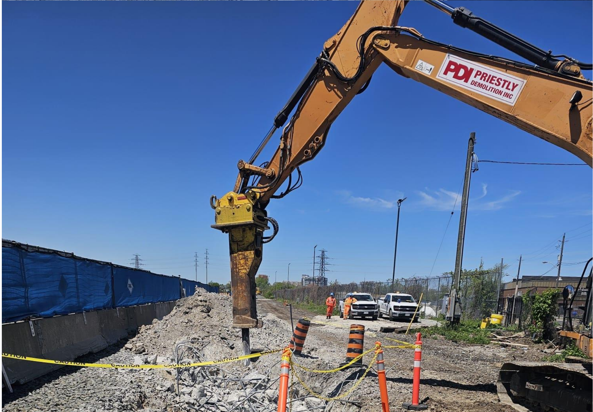
Retaining wall and signal footing demolition (in-corridor)
